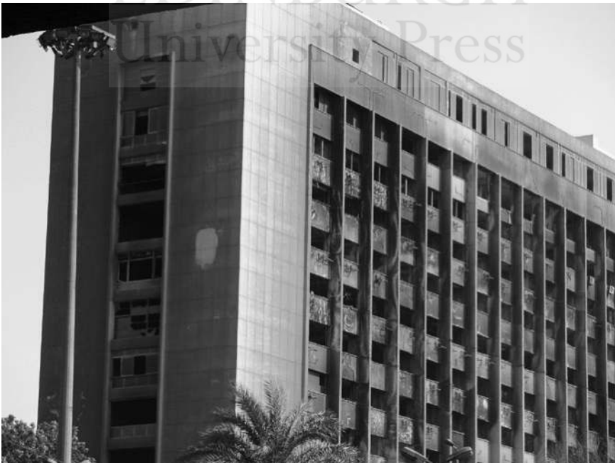
Figure 2.2 Ministry of Interior building, Cairo. Photo: Deborah L. Wheeler, March 2013.
