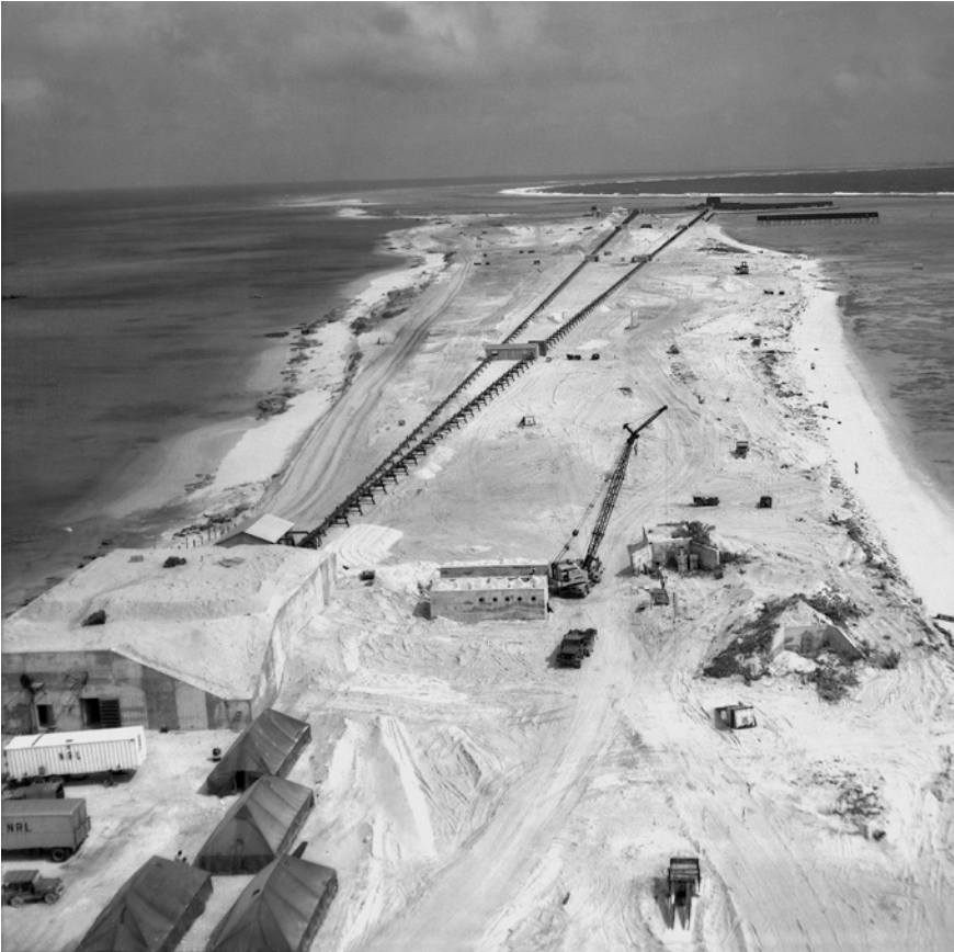
Figure 2. Looking north on Runit Island in April 1956 at preparations for the May 5 Operation Redwing Lacrosse nuclear test. The concrete structure in the middle left is Scientific Station 1310, an Alpha Recording Station. In the upper right is Station 24 at ground zero. A steel pipe array leads from Station 24 back to the Station 1310, providing a vacuum environment for neutron measurements.
