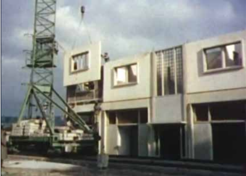
Figure 6.3. Prefabricated elements speed up the building process. Film still from Somewhere to Live (dir. Jacques Brunius, ECA, 1951).
