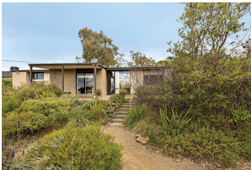
Figure 9.3: 3 Anstey Street, Pearce, the mid-century modern Gascoigne home designed by architect Theo Bischoff.
