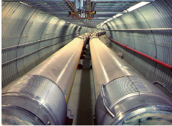
Fig. 9.5 In RHIC tunnel at the Brookhaven National Laboratory [2]. The two rings of the 255 GeV polarized proton beams and heavy ion collider run parallel over 3.8 km, and intersect at two experiments, STAR and SPHENIX
