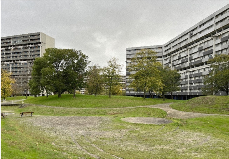
Fig. 1. The Messenger and Poulenc buildings and the natural public space threatened with demolition, Toulouse Le Mirail, 2023 (Photograph by Adam W. Pugliese, 2023).
