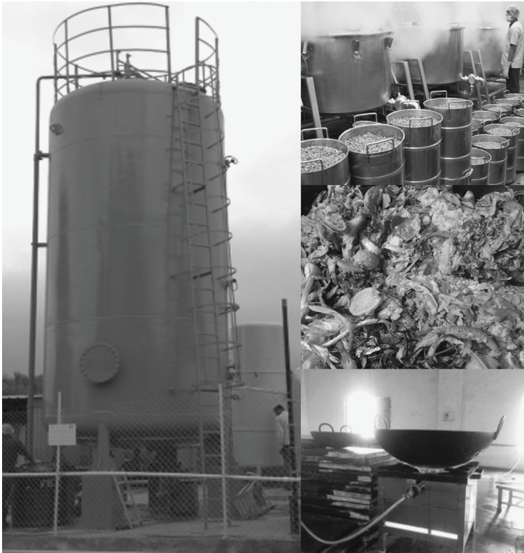
FIGURE 3.1 Biogas plant at Bellary in Karnataka State for the generation of biogas and bio manure from food waste.
