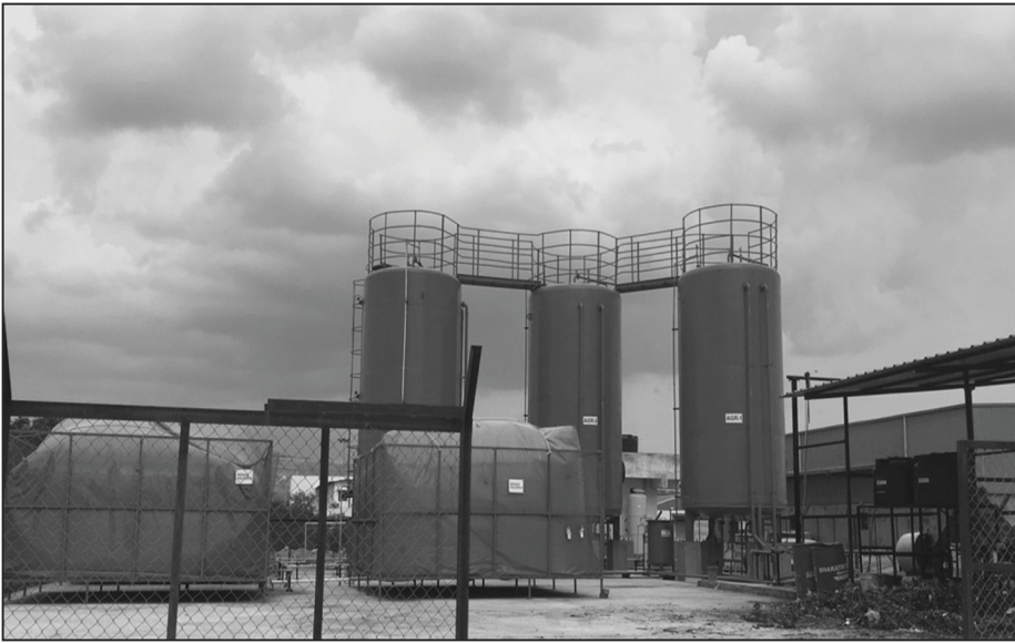
FIGURE 3.2 A 5 TPD biogas plant for the generation of biogas based off-grid power and bio manure from organic fraction of MSW and leachate.
