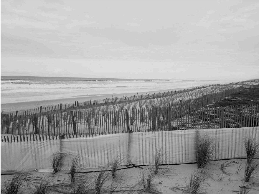
Figure 11.1 Marram plantings to reinforce the foredune at Lacanau Ocean, France, 2022 Source: Photo by J.G. Freitas
