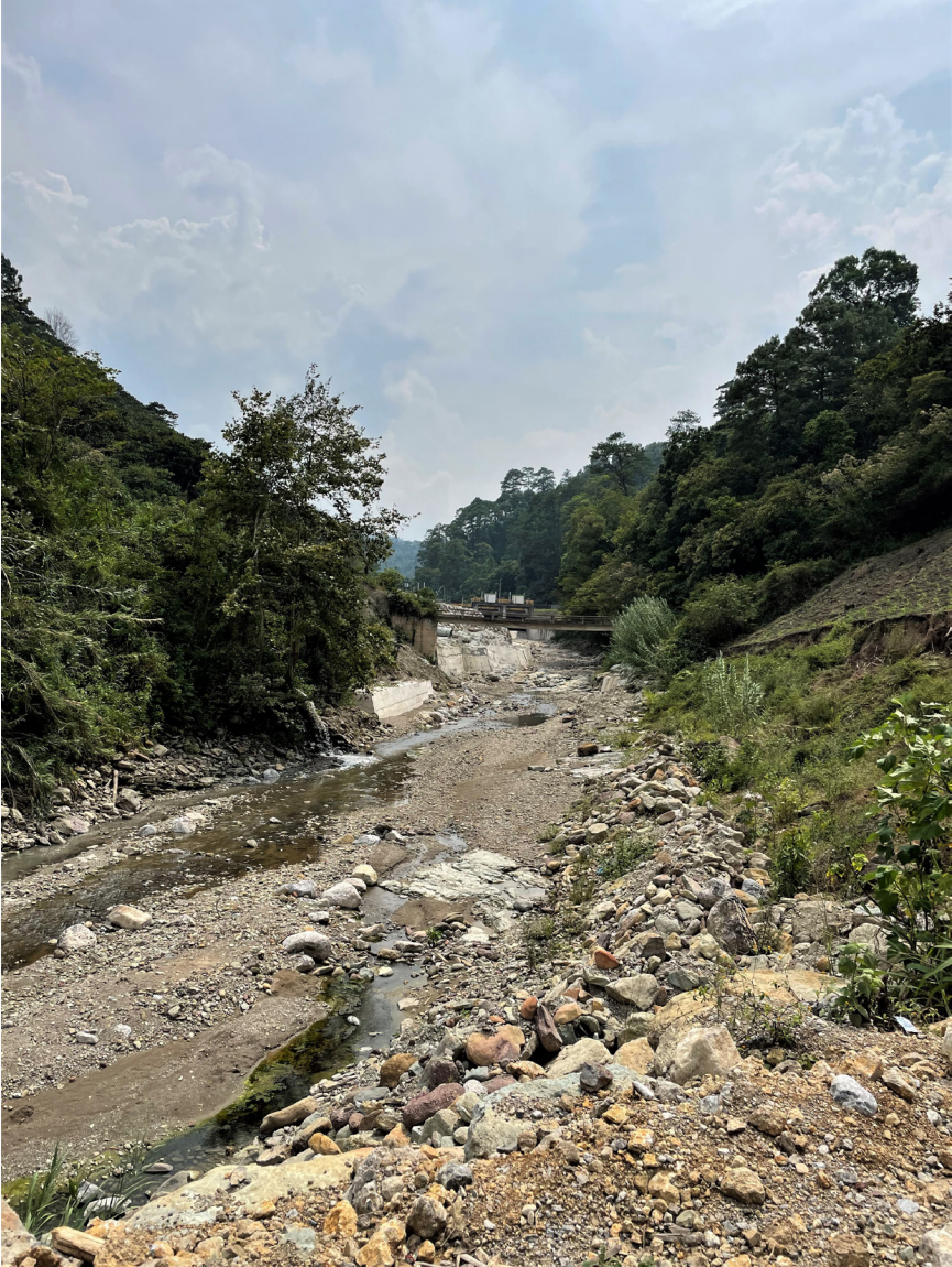
FIGURE 14. Cotzal River after passing through one of Enel's diversion dams, which diverts the river into a concrete channel, leaving the riverbed dry, May 2022. Photo by author.
