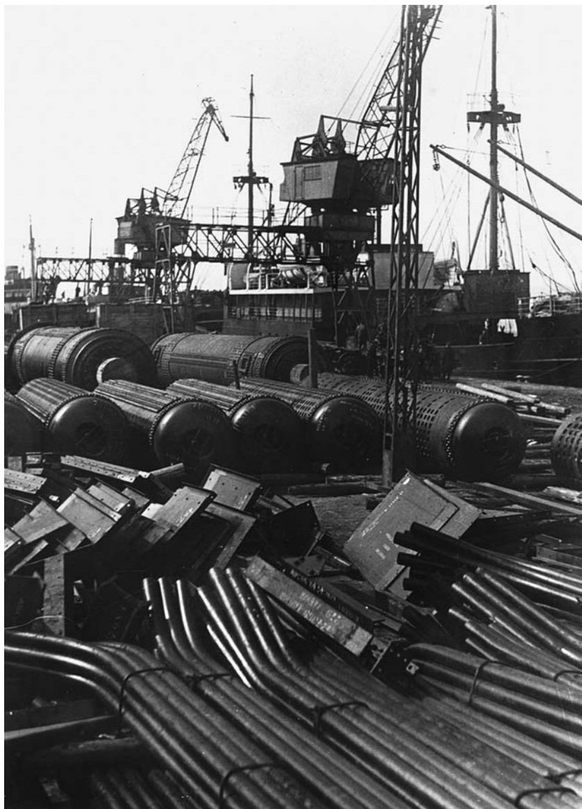
PLATE 27. Valuables bought through Torgsin paid for imports during the first five-year plans. Industrial equipment imported from the United States. Leningrad port, 1931 (RGAKFD).
