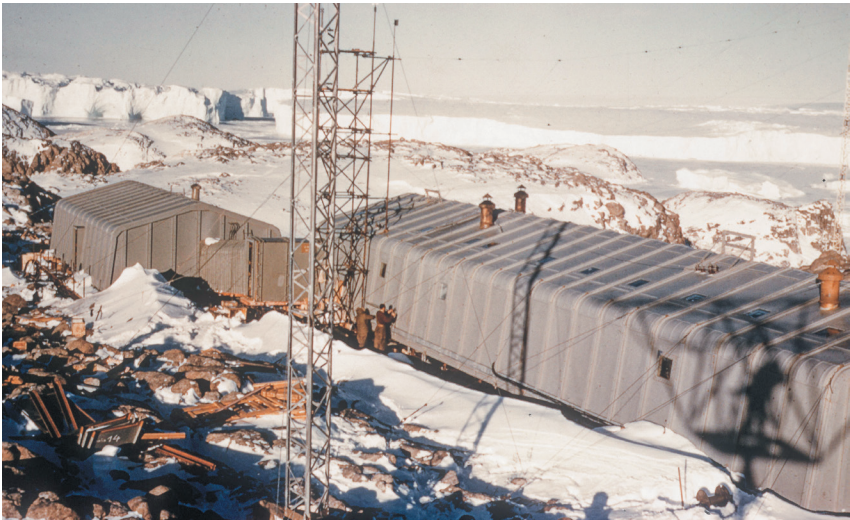
FIGURE 13. The first two buildings for the Dumont-d'Urville base, built for the International Geophysical Year, 1956 (Archipôles, IPEV).
