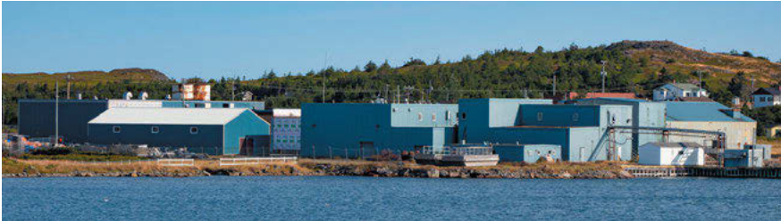
Abandoned fish processing plant in Catalina.
