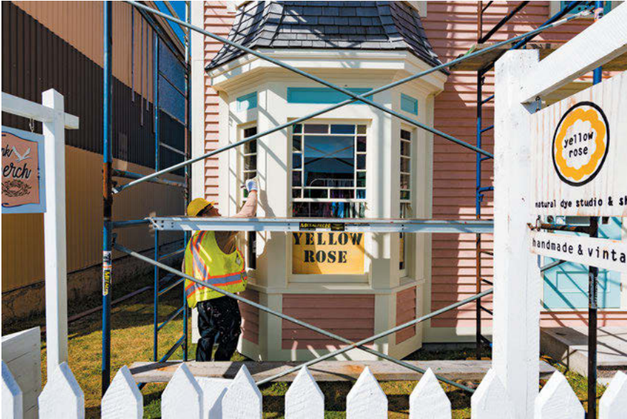
Plate 84: The renovated Levi Templeman house, being painted by Todd Way.
