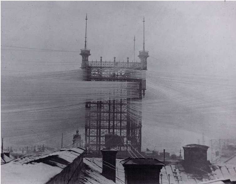
Figure 1: A Stockholm tower connecting 5,000 telephone lines at the end of the nineteenth century. 2
