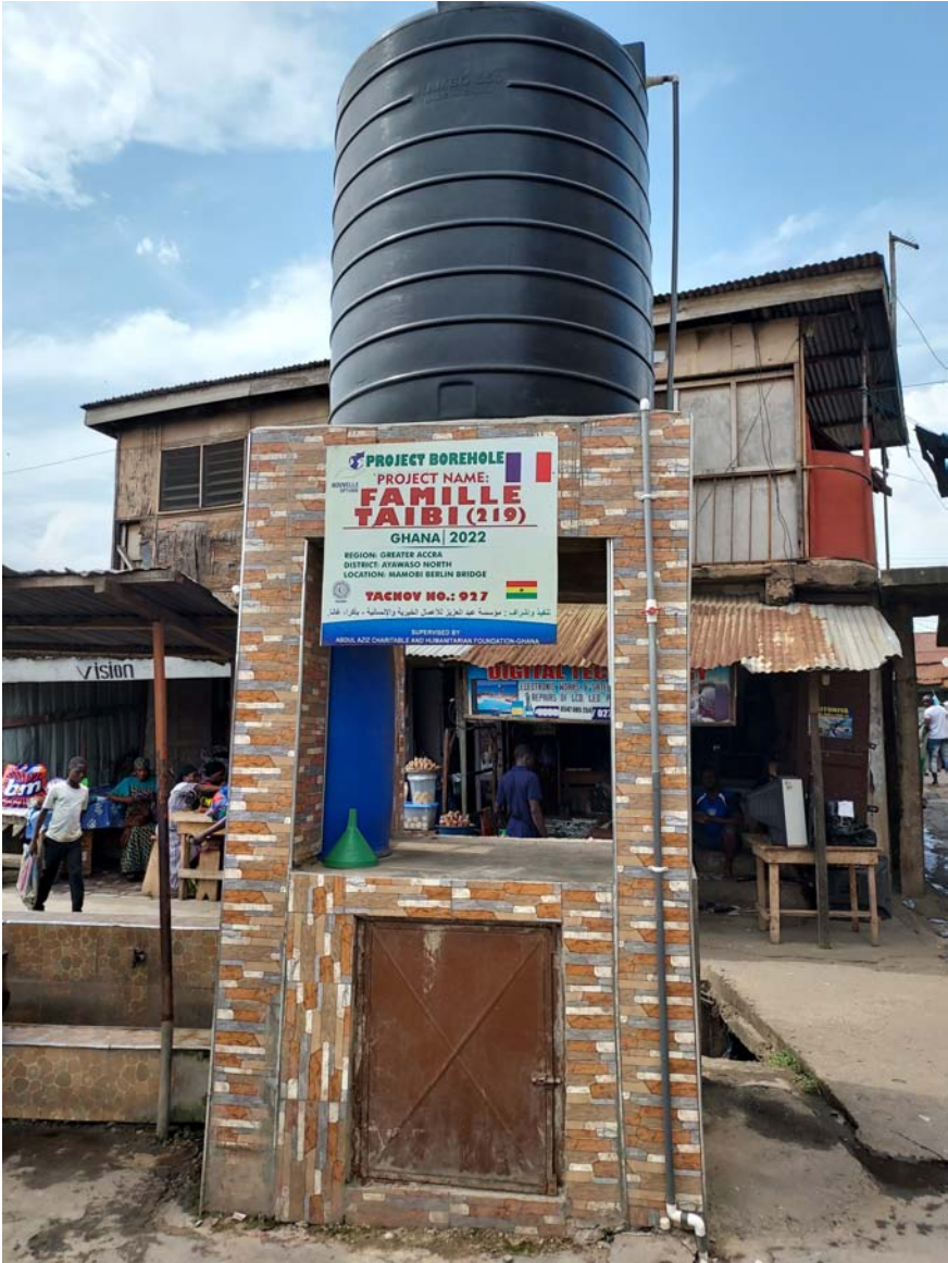
FIGURE 23 Nouvelle Optique borehole in Mamobi, Accra. Supervised by Abdul-Aziz Charitable and Humanitarian Foundation PHOTO: HOLGER WEISS/2022
