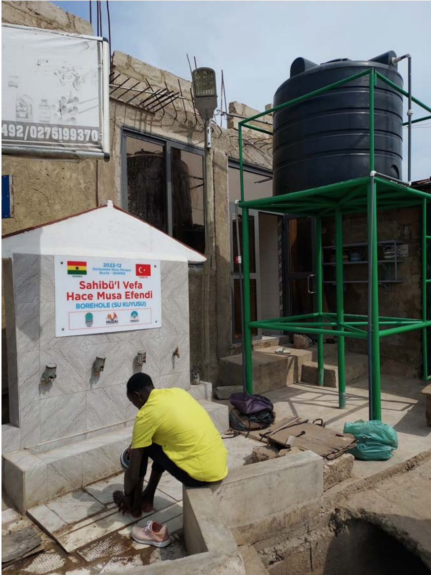
FIGURE 20 HUDAI borehole in Nima, Accra PHOTO: HOLGER WEISS/2022
