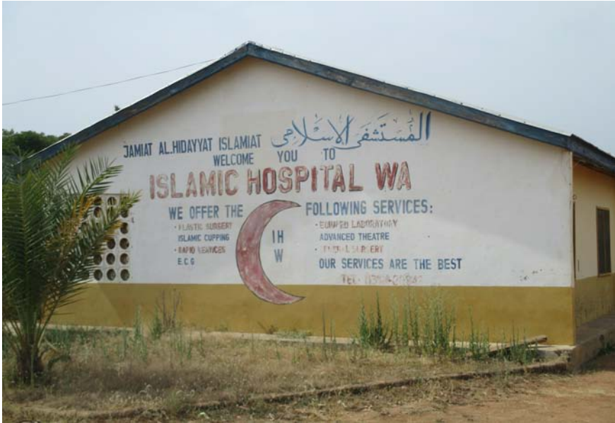
FIGURE 35 Islamic Hospital Wa PHOTO: HOLGER WEISS/2019
