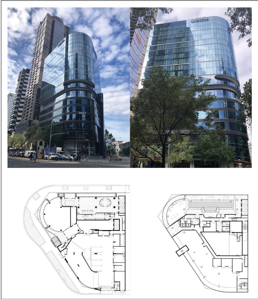
Fig. 8.8 Pictures and floorplans of an existing building extension with a timber structure
