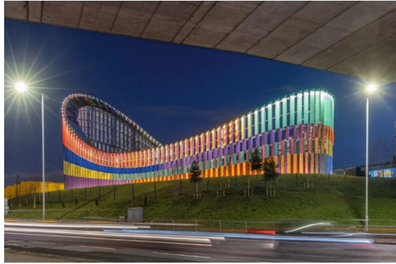
Fig. 5.5 Brent Cross Town primary substation [43]
