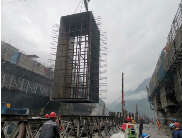
Fig. 6. Adjustment of the initial installation section in place
