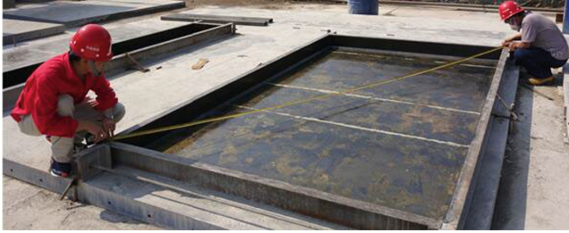
Fig. 13. Formwork assembly verification
