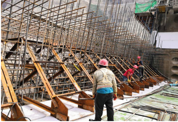
Fig. 16. Installation of pre-fabricated bracket formwork on site
