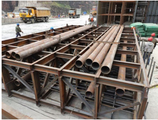
Fig. 7. Overall assembly of steel lining and embedded truss
