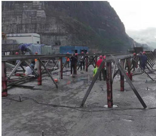
Fig. 5. Installation of supporting track
