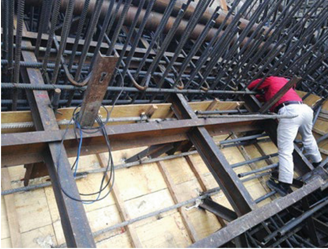
Fig. 8. Installation of bottom formwork for supporting beams
