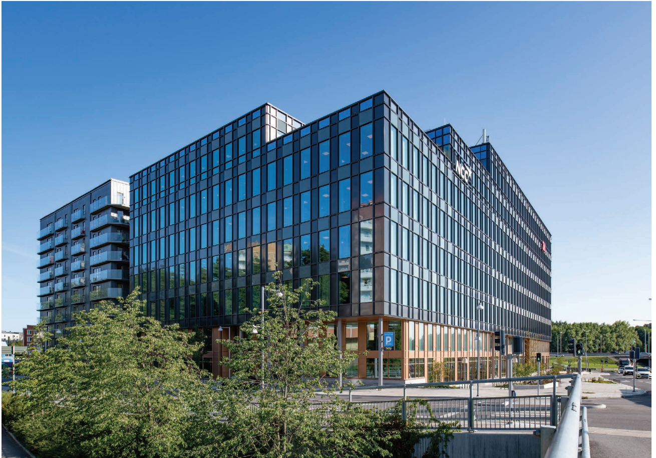
Figure 5.112 Pedestrian view of NCC Headquarters. Credits: White Arkitekter AB.
