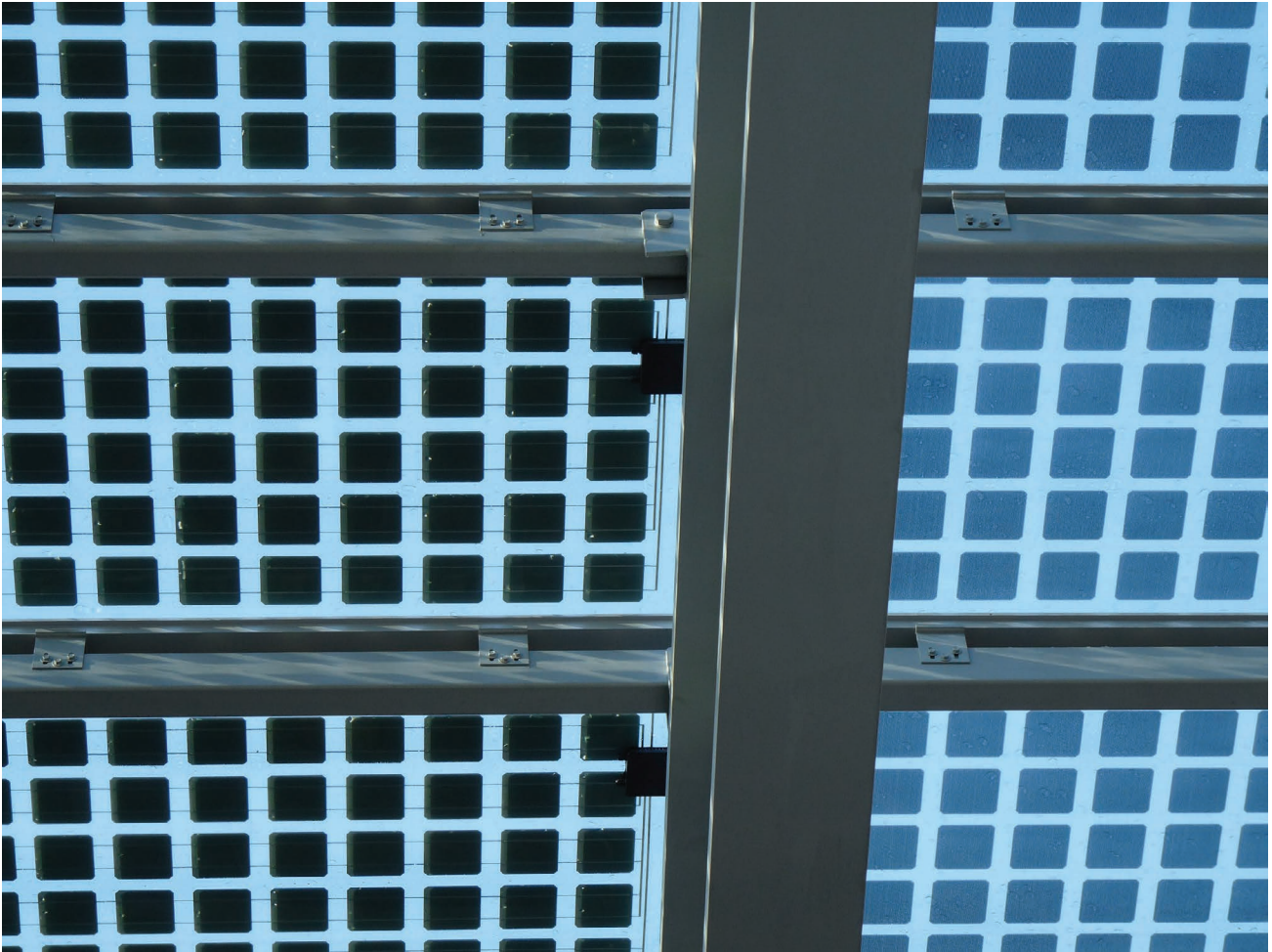
Figure 5.62 Detail of the BIPV skylight and dummy modules. Credits: Francesco Frontini, SUPSI.
