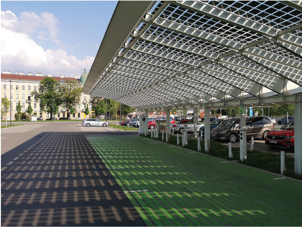
Figure 5.135 BIPV car canopy at the arrival centre in Schönbrunn. Credits: Francesco Frontini, SUPSI.
