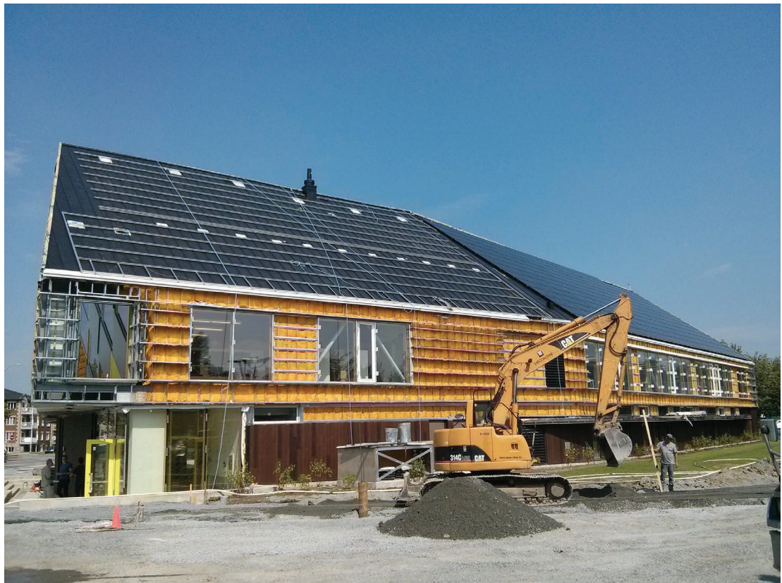
Figure 5.4 Varenes library under construction. Credits: Jose Candanedo.
