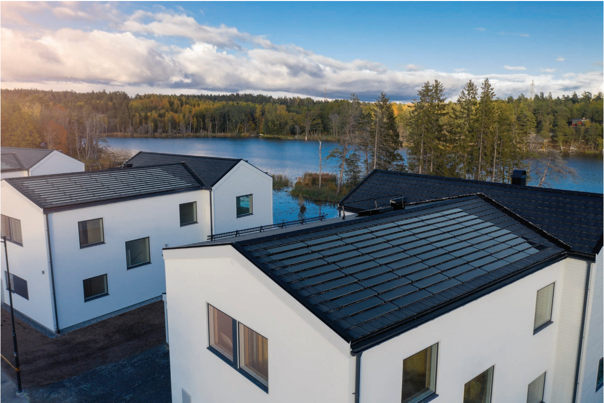
Figure 5.27 Close-up view of the Glasberga BIPV roofs. Credits: Soltech Energy Sweden.
