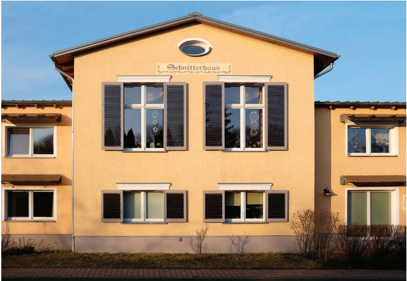
Figure 3.15 Residential building in Nechlin, Germany, with “Solar Window Shutters” designed and patented by Astrid Schneider. Photo: Astrid Schneider, Solar Architecture, Berlin.
