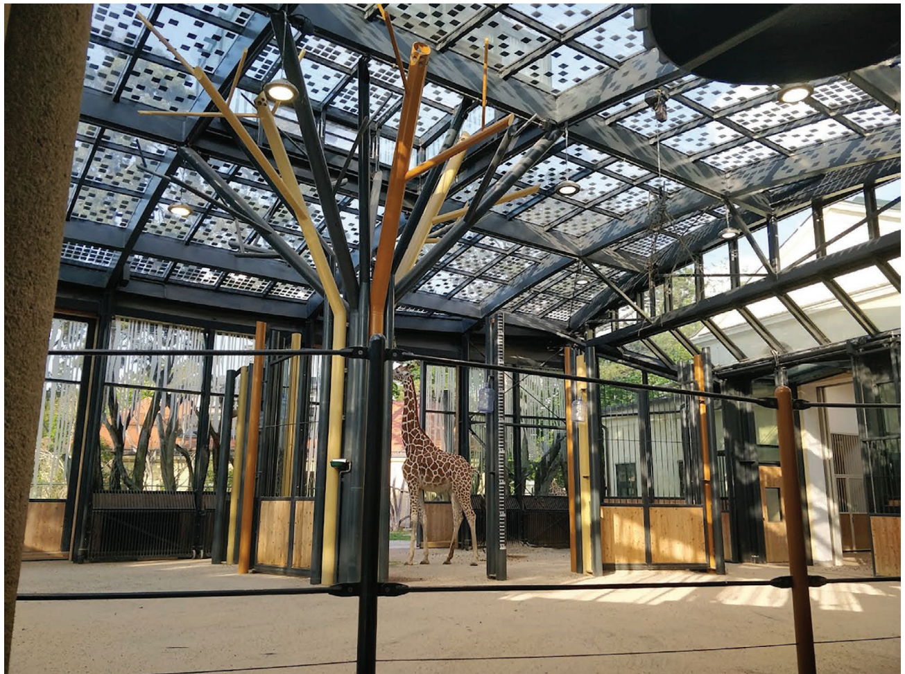
Figure 3.5 BIPV skylight at the Schönbrunn Zoo, in Vienna, using customised solar cell patterns. Photo: Costa Kapsis.
