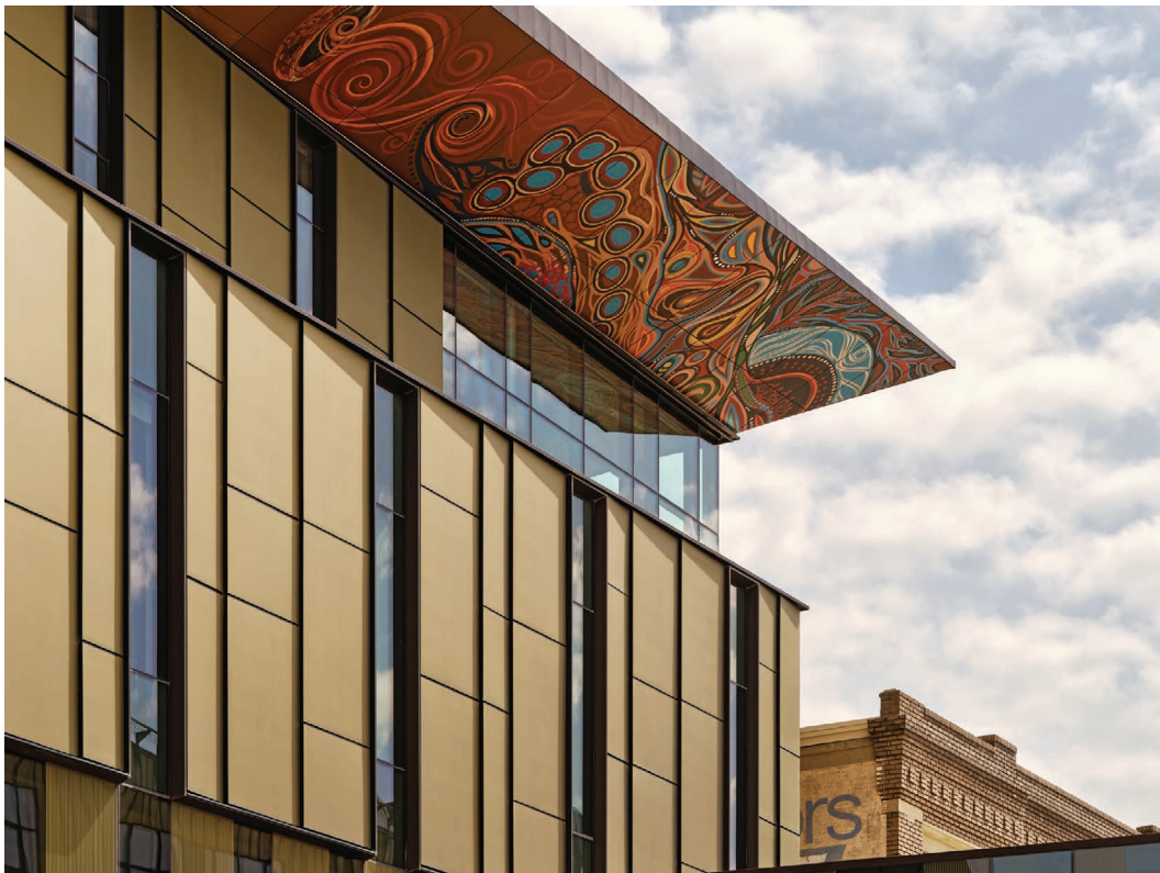
Figure 5.85 BIPV rainscreen detail of Manitou A Bi Bii Daziigae University building. Credits: Diamond Schmitt Architects.
