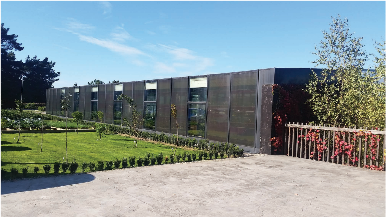
Figure 5.50 Semitransparent curtain wall at the Azurmendi Restaurant. Credits: Onyx Solar.
