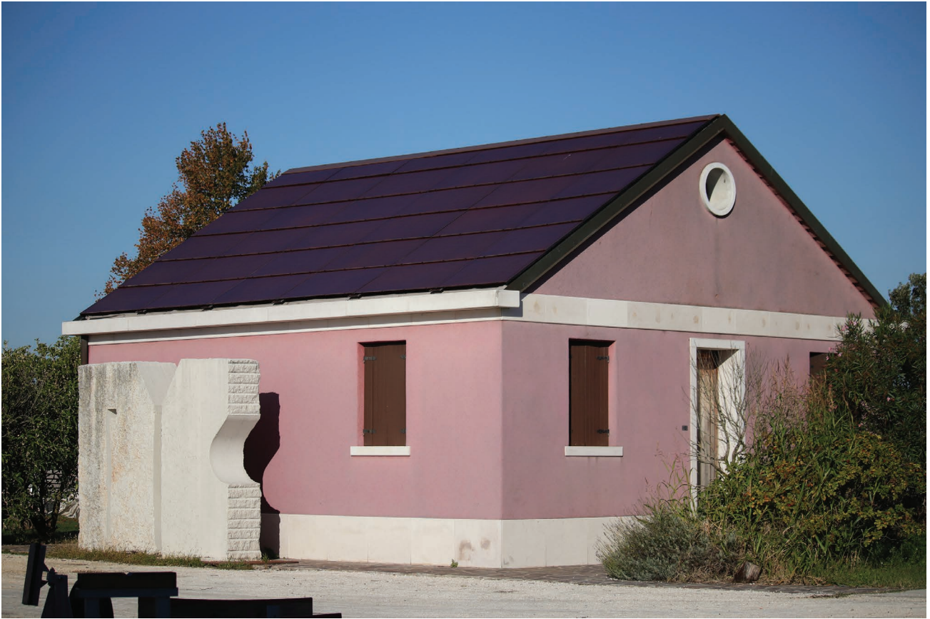
Figure 5.36 BIPV roof in a heritage building at the Urban Park in Certosa Island. Credits: GruppoSTG.
