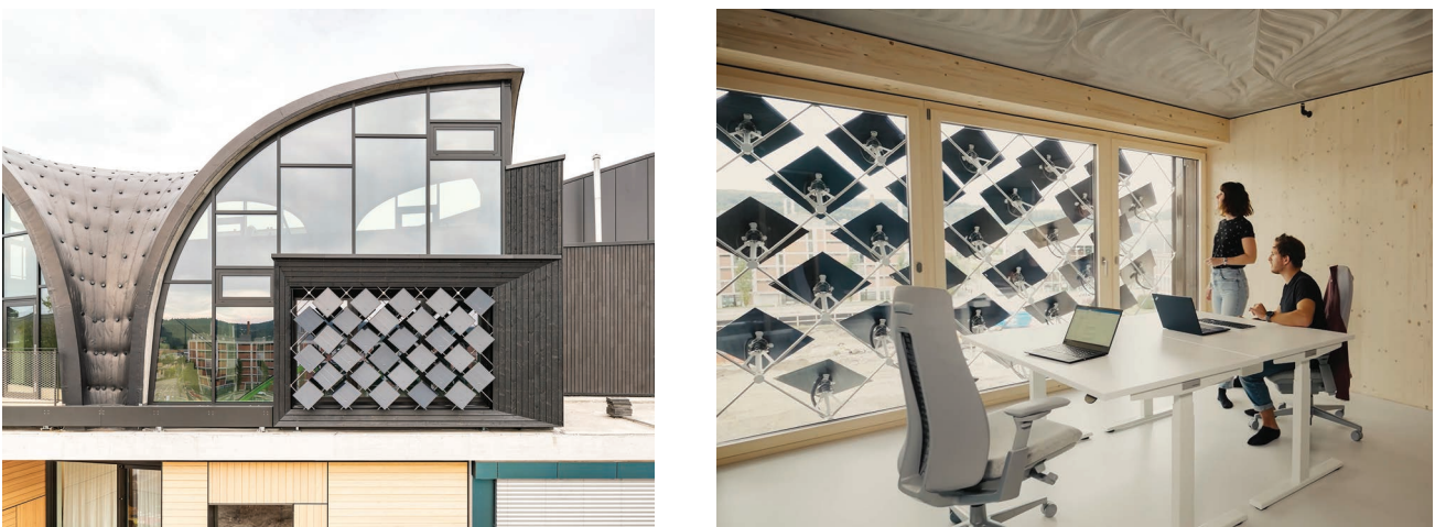
Figure 3.14 The movable BIPV solar shading system, Solskin, installed at HiLo, NEST building, in Dübendorf. Photos: courtesy of Roman Keller (left) and Chair of Architecture and Building Systems (A/S) Group (right).
