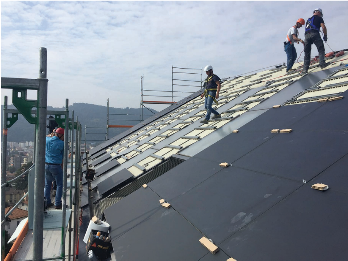
Figure 5.80 DeltaROSSO BIPV ventilated roof under construction. Credits: Isa Zanetti, SUPSI.
