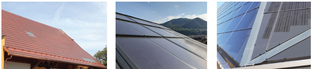
Figure 3.6 Left: Renovation featuring terracotta BIPV roof tiles on a historic farm in Ecuwillens, Canton of Fribourg, Switzerland; middle: solar shingles in a discontinuous roof; right: special roof parts for the Umwelt Arena in Spreitenbach, Switzerland. The modules are in an “all black” appearance with a black backsheet and covered interconnectors between the cell strings. Architect: Rene Schmid. Photos courtesy of Patrick Heinstejn, CSEM (left) SUPSI; Flisom-Schweizer (middle); P. Bonomo (right).
