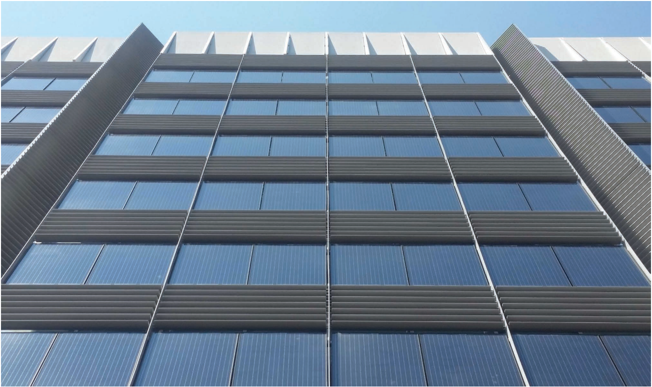
Figure 5.102 Close-up of the Palazzo Argonauta BIPV rainscreen. Credits: DiARC.
