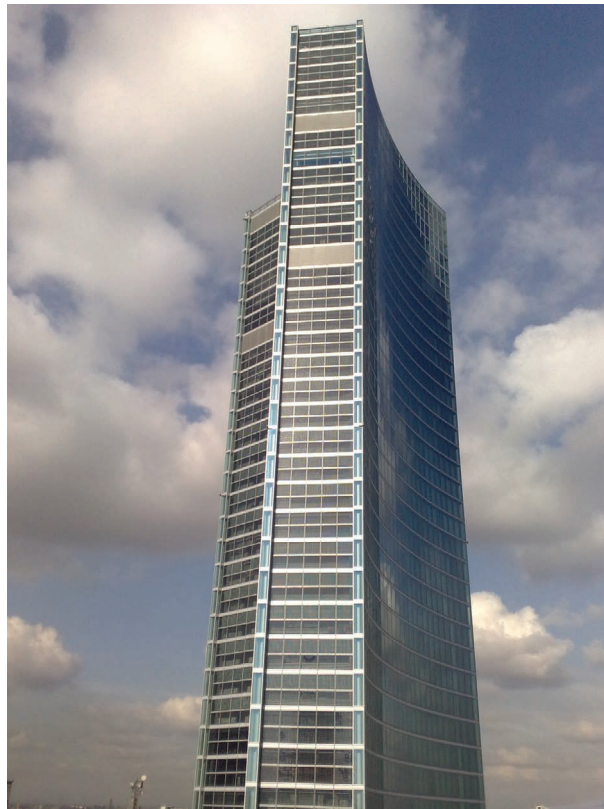
Figure 5.118 BIPV unitised curtain wall façade at Palazzo Lombardia. Credits: DiARC.
