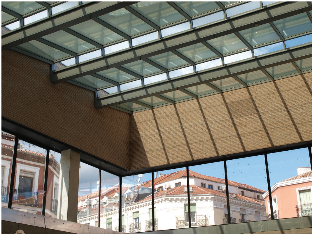
Figure 5.43 Interior view of the BIPV skylight at San Antón Market. Credits: Onyx Solar.
