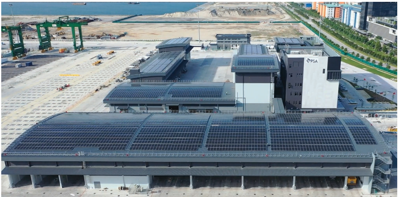
Figure 5.74 Eagle-eye view of the Tuas Port building complex. Credits: PSA.
