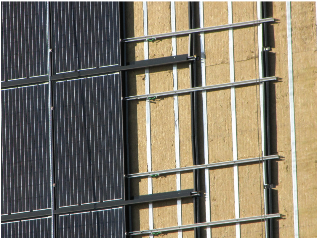
Figure 5.68 Detail of the BIPV rainscreen at Jeanne & Peter Loughheed Performing Arts Centre. Credits: Gordon Howell, HME.
