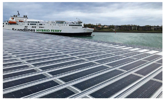
Figure 3.7 Flat inclined roofs of the company “Trumpf” in Germany at the Rostock harbour. The crystalline solar cells are integrated into plastic laminates, incorporated in aluminium sheet roofing. The PV modules' weight is less than 4 kg per m 2 . Picture: DAS Energy Ltd., Wiener Neustadt, Austria.
