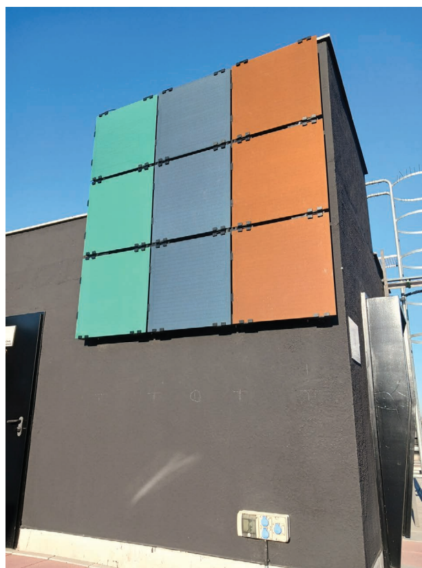
Figure 2.1 Coloured demonstration façade at CIEMAT, Spain. In this example, green and terracotta BIPV modules reduce the efficiency by 4% and 15%, respectively, when compared to the anthracite colour. Ref: RINGS-BIPV project, 2023. Source: N. Martín-Chivelet, CIEMAT.
