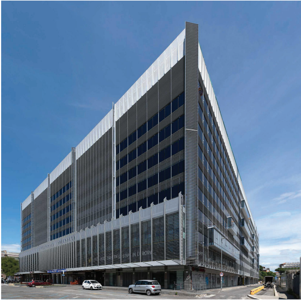
Figure 5.100 Pedestrian view of the renovated Palazzo Argonauta. Credits: DiARC.
