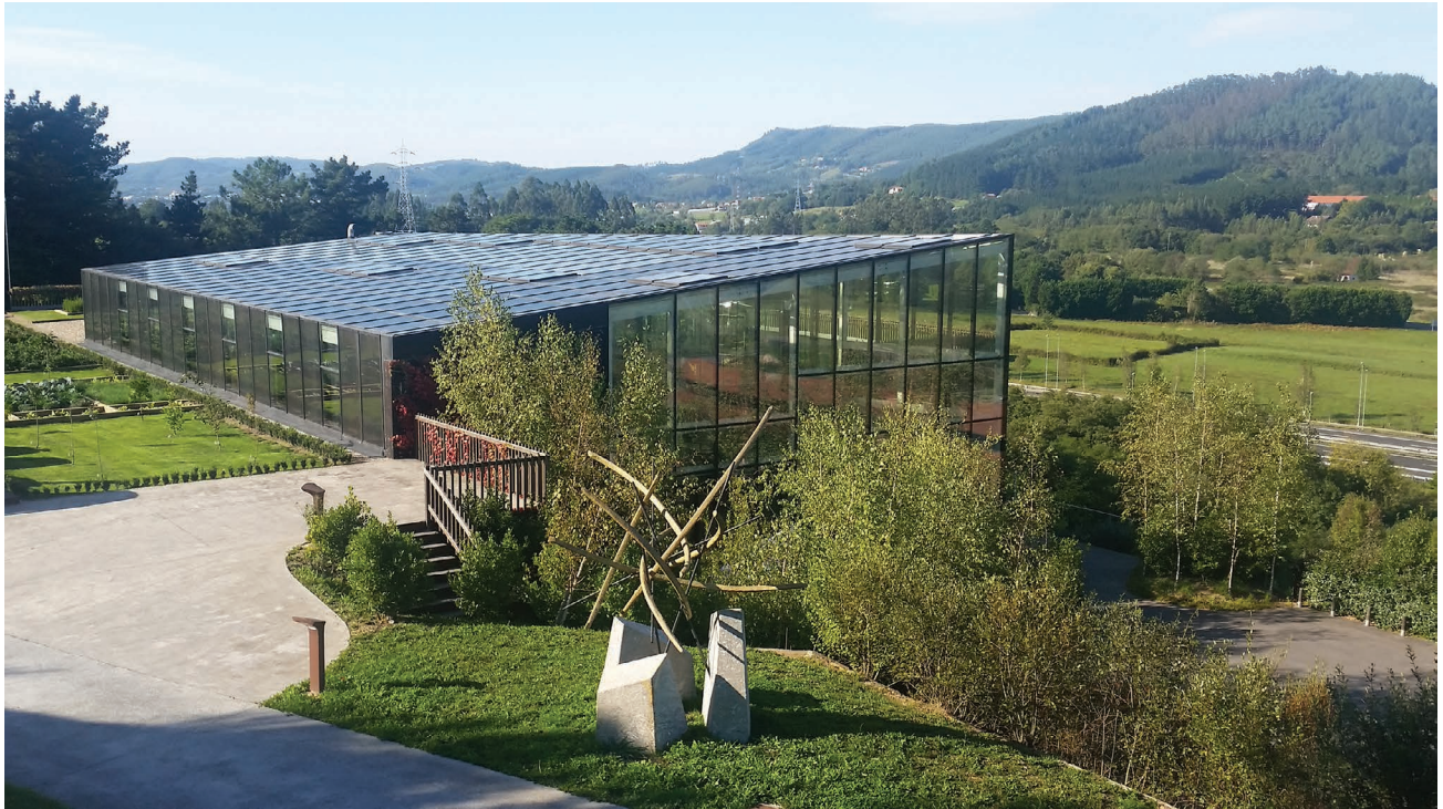
Figure 5.48 General view of Azurmendi Restaurant showing the BIPV façade and skylight. Credits: Onyx Solar.
