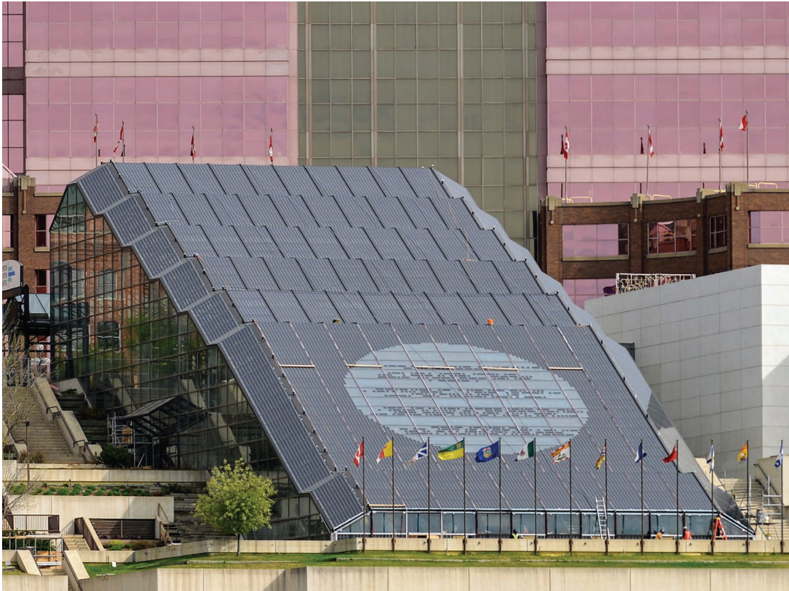
Figure 5.54 General view of Edmonton Convention Centre. Credits: Onyx Solar.
