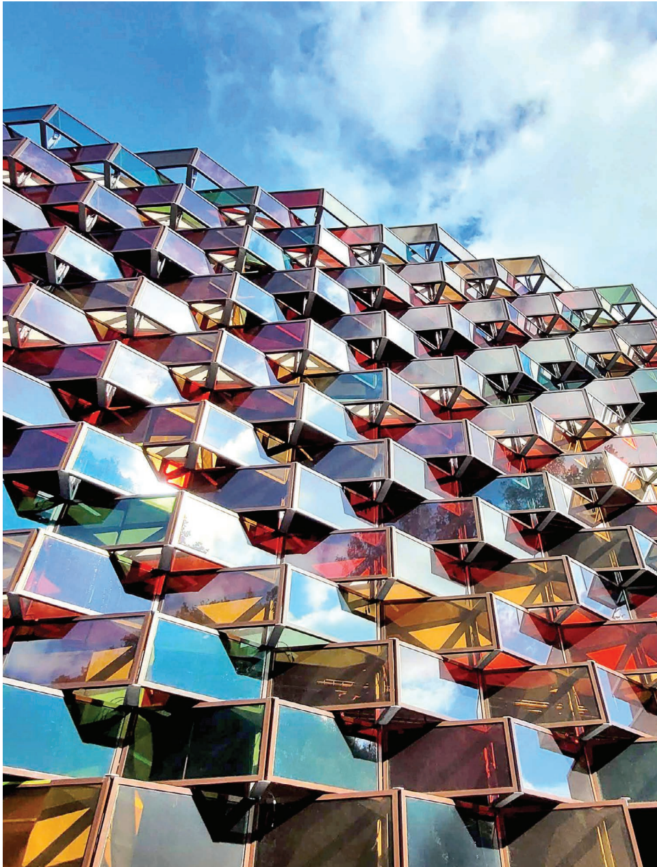
Figure 5.124 Coloured transparent BIPV shading at Gothenburg Garage. Credits: Soltech Energy Sweden.
