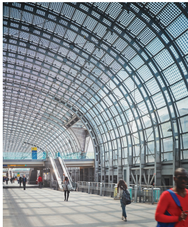
Figure 5.61 Pedestrian interior view of the BIPV skylight at Porta Susa AV Station. Credits: Julien Lanoo.
