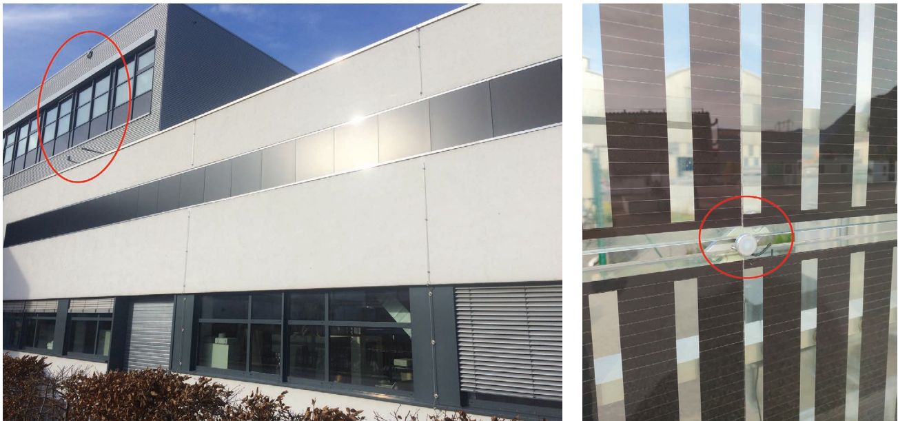
Figure 6.1 Two examples of solar radiation sensors location: on the plane of a BIPV façade (left) and integrated into a BIPV module, developed under the BIPV Boost project (right).
