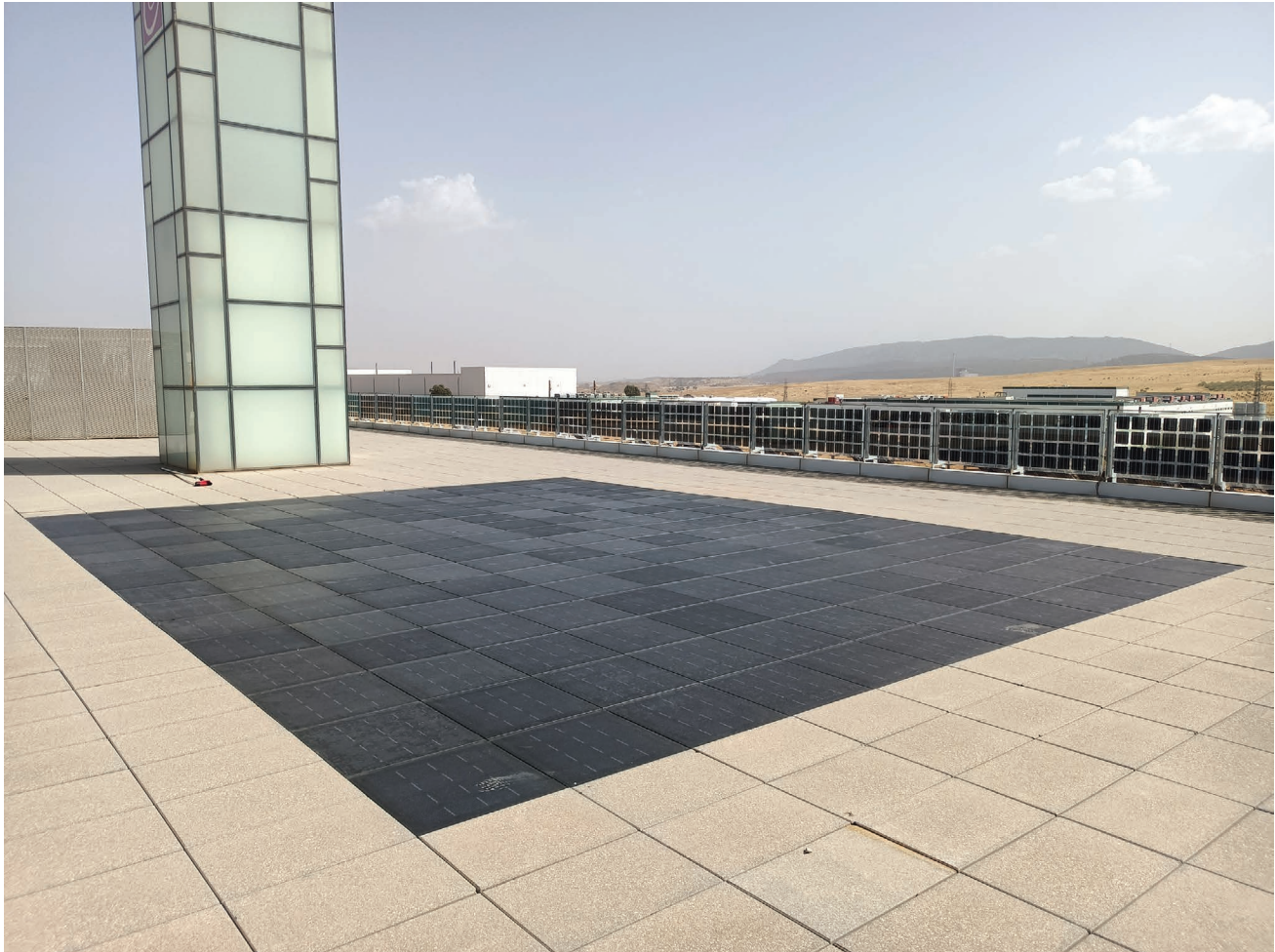
Figure 3.8 Walkable BIPV floor and balustrade realised with laminated safety glass and c-Si solar cells. Source: BIPVBOOST.
