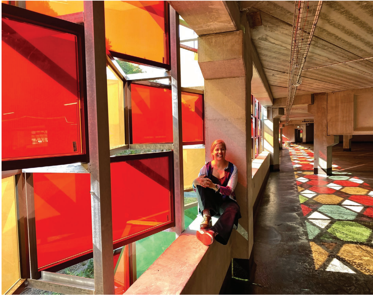
Figure 5.125 Detail from the interior of Gothenburg Garage. Credits: Soltech Energy Sweden.
