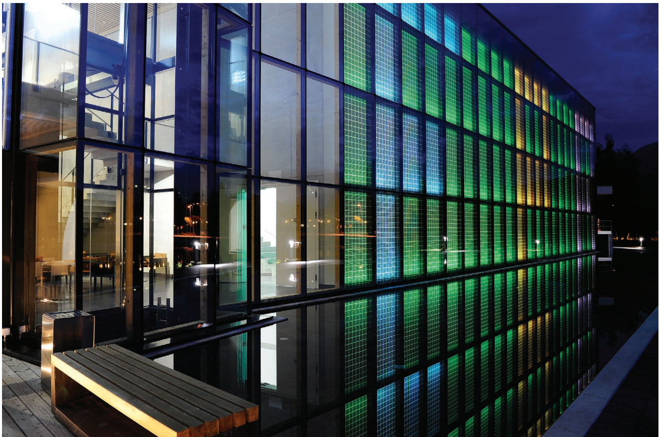
Figure 2.9 Night view of the BIPV curtain wall of Pierre Arnaud artwork gallery in Lens, Switzerland, showing coloured LED projections. Designed by: architect Jean-Pierre Emery. Credits: Ertex Solar.
