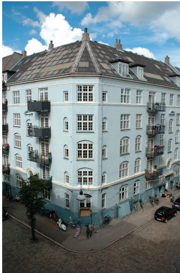
Figure 5.31 Andreas Bjørns St.1 before renovation. Credits: Solar City Denmark.
