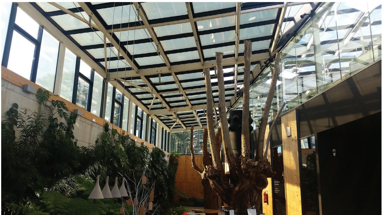
Figure 5.49 Interior view of BIPV curtain wall and skylight at the Azurmendi Restaurant. Credits: Onyx Solar.
