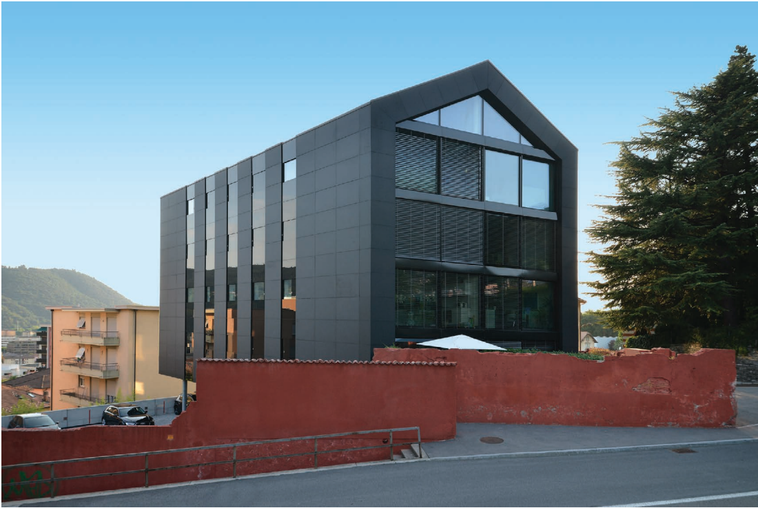
Figure 5.78 Pedestrian view of DeltaROSSO building. Credits: Isa Zanetti, SUPSI.
