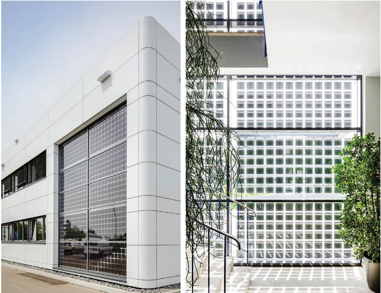
Figure 3.13 Semi-transparent thermally insulated BIPV façade in an office building. Photo: Sunovation GmbH, Germany.
