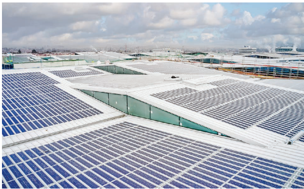
Figure 3.7 Flat inclined roofs of the company “Trumpf” in Germany at the Rostock harbour. The crystalline solar cells are integrated into plastic laminates, incorporated in aluminium sheet roofing. The PV modules' weight is less than 4 kg per m 2 . Picture: DAS Energy Ltd., Wiener Neustadt, Austria.
