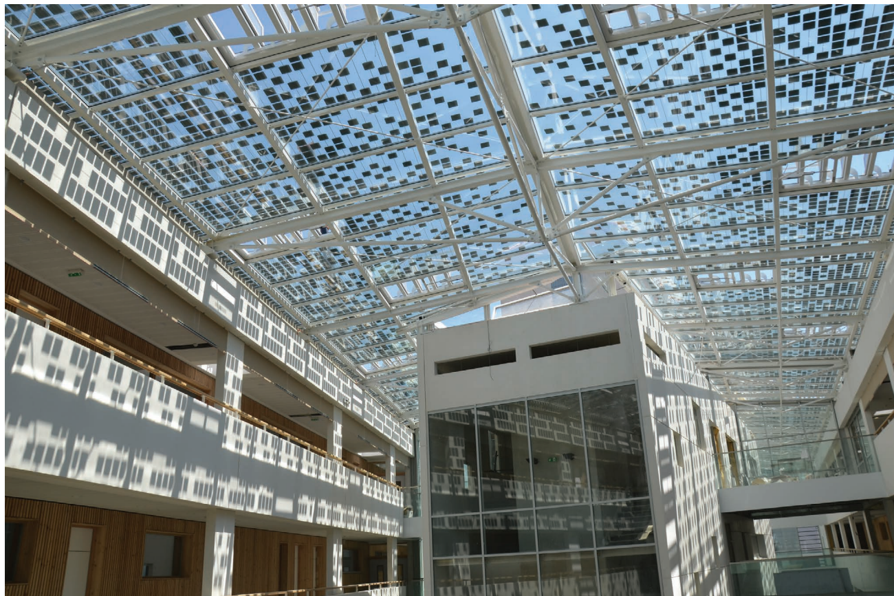
Figure 2.4 Semi-transparent BIPV skylight using c-Si solar cells at a school, in Courbevoie, France. Photo credits: MTECH & CSTB.
