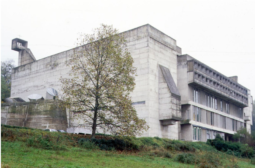
Fig. 23.9 The Dominican monastery of Sainte-Marie de La Tourette (1954–60). On the right, undulating glass walls; to the left, the curved volume and the “light cannons” that bring light into the crypt. Photo by author (1999), CC BY-NC-ND.
