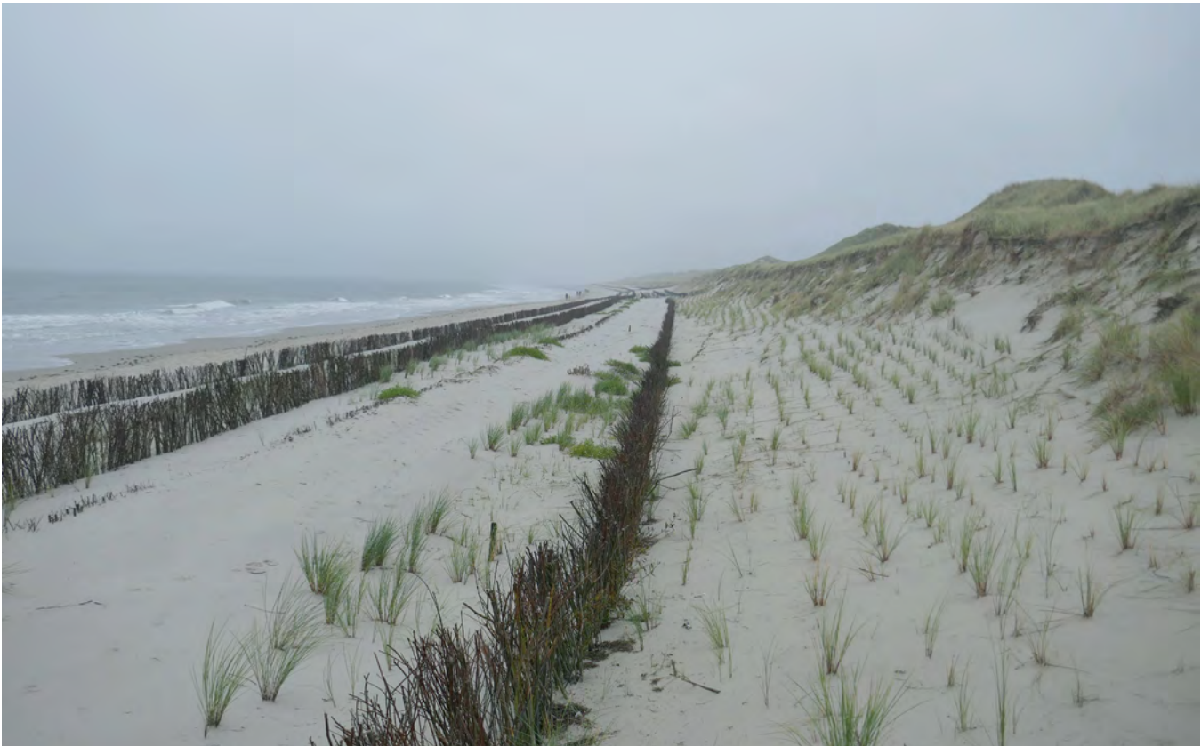
Figure 5.8: Amrum, Germany: Fresh stalk plantings and sand trapping fences to secure and further build up the coastal dunes that protect the island of Amrum, Germany. Photo: Philipp Jordan.
