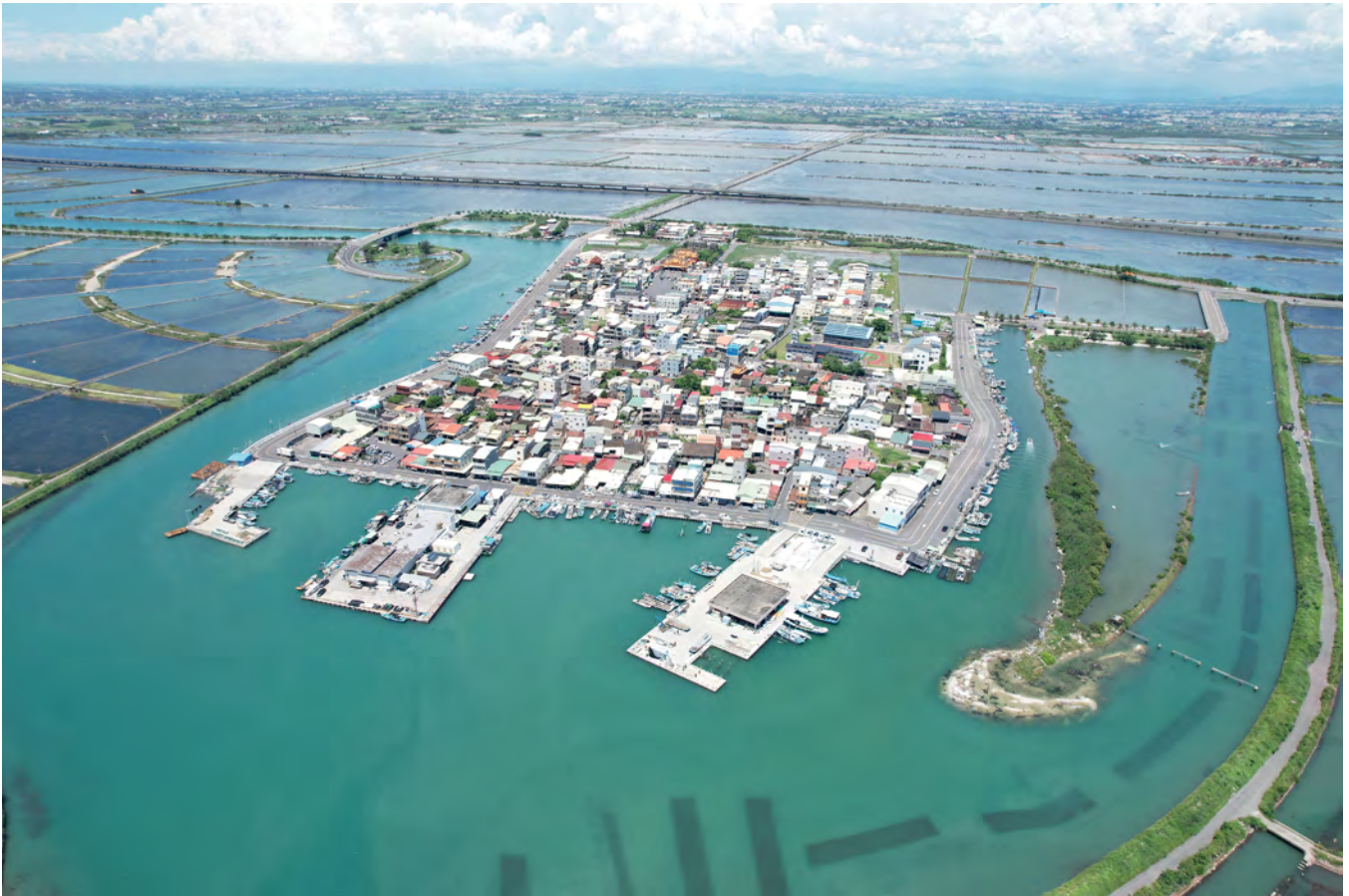
Figure 5.10: Tainan, Taiwan: A typical coastal community in Tainan protected by a sea dike with protection level of 50-year storm surge, air-drone photo, Taiwan. Photo: Hsiao-Wen Wang.
