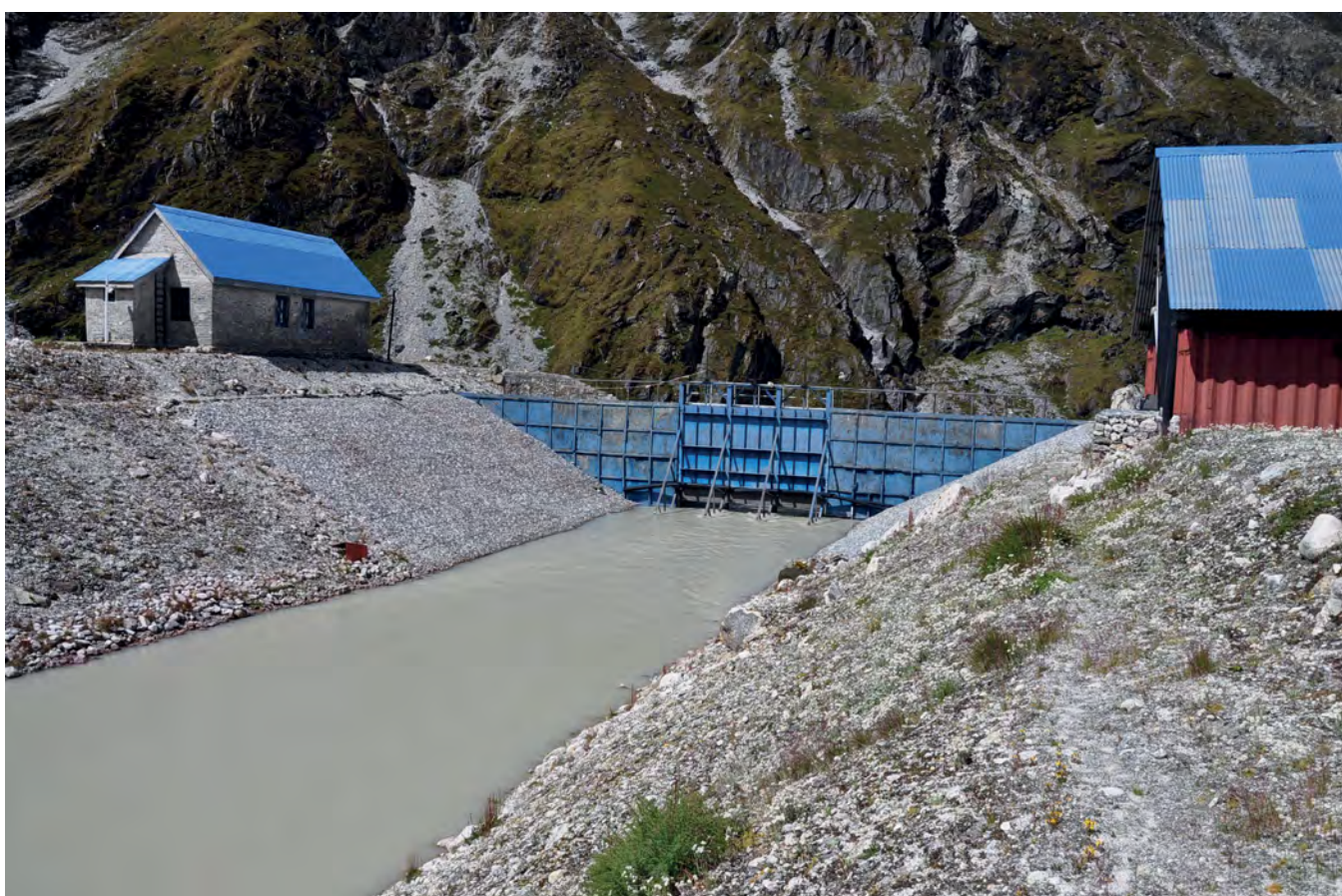
Figure 5.6: Lake Tsho Rolpa, Nepal: Artificial outlet of the Tsho Rolpa lake to reduce the pressure on the moraine dam, Nepal. Photo: Udo Schickhoff.
