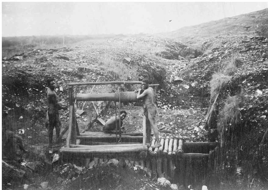
Figure 4.6 Shaft sinking with a windlass, 1901–6 Source: FHA, PC, VKK871:133.
