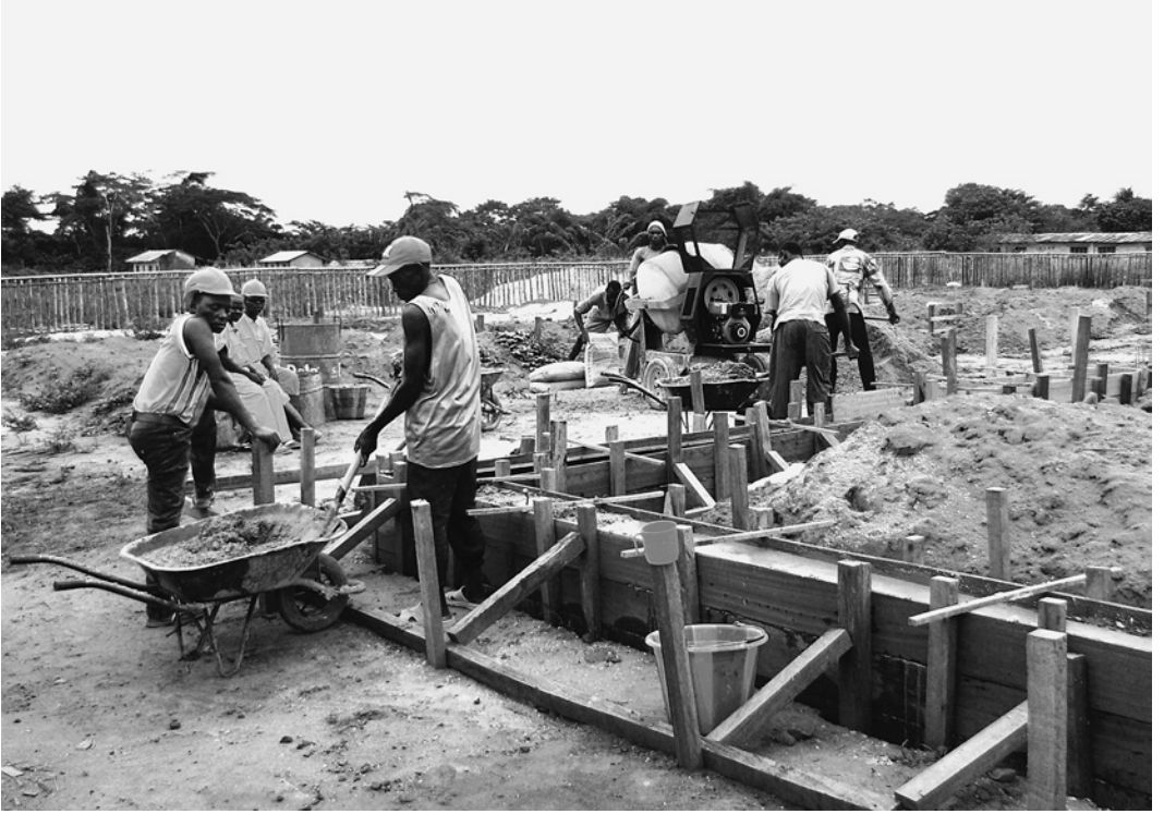
CTI workers building a school in Mombwassa
