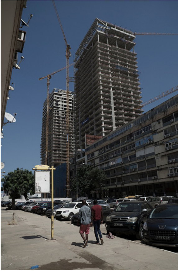
Figure 4.1. View of Kinaxixe Square in 2015 after the destruction of Kinaxixe Marketplace. Source: Rui Sérgio Afonso.
