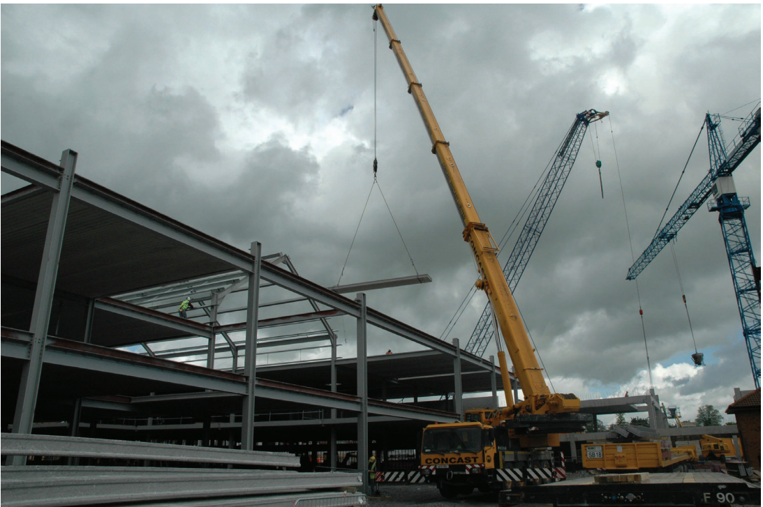
Figure 4-15. Cranage on the building site during construction.
