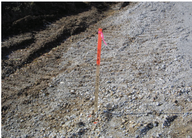
Figure 5-7. Offset stake and color code ribbon.
