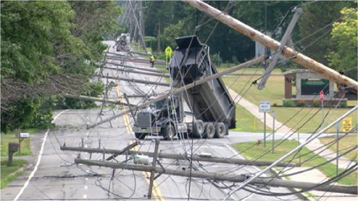
Figure 3-8. Dump truck gets tangled in power lines, pulls down 12 utility poles outside Rush-Henrietta High School in upstate New York (July 24, 2018) WFLA ABC Affiliate.
