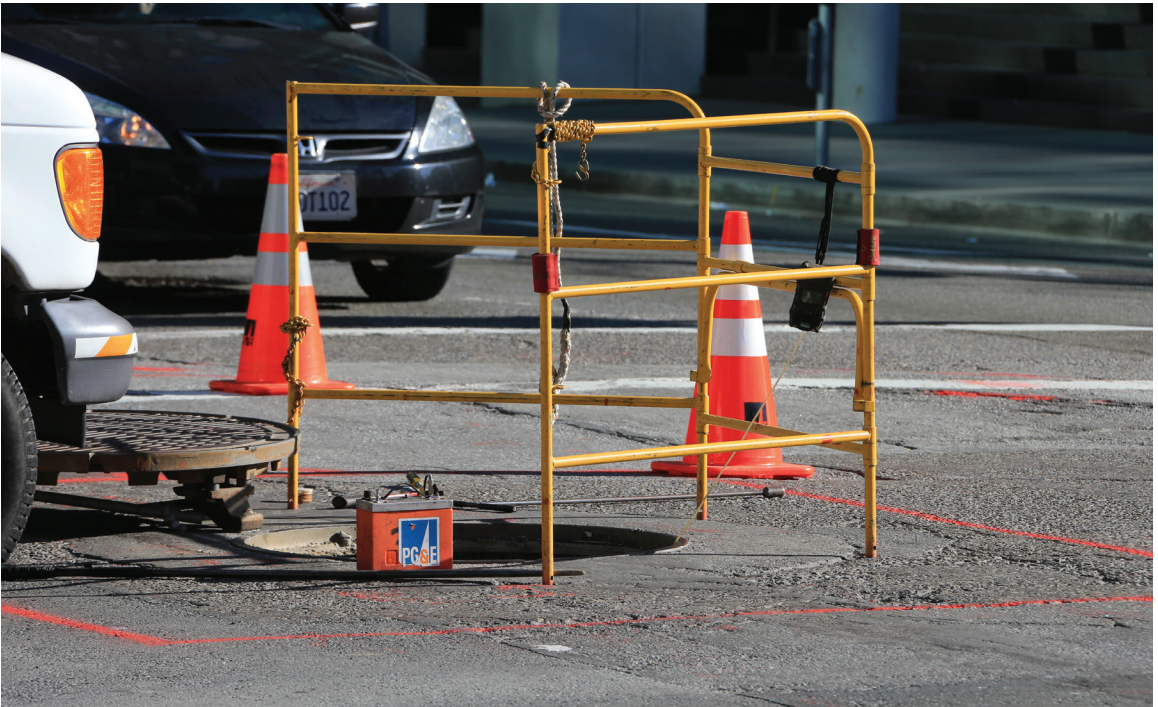
Figure 11-7. A gas-monitoring device in use at a manhole entry.
