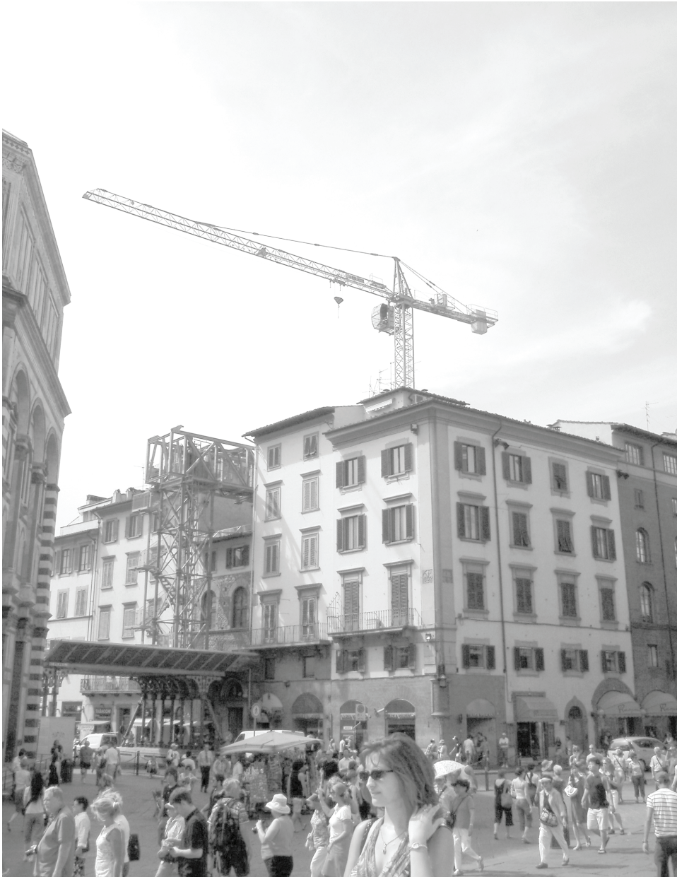
Figure 1-1. Highly restricted work sites adjacent to buildings, as shown in this image from Florence, Italy, can require elaborate and costly scaffolding for access. The planning and permitting for such temporary works are seldom trivial.
