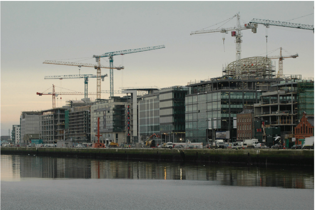
Figure 4-14. The building site during construction.
