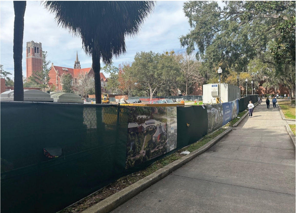
Figure 3-16. Construction activity on the campus of the University of Florida, Gainesville, FL. This walkway must be maintained with full accessibility to ensure the safety and effective flow of faculty, staff, and students through campus (Source: Author, 2024).
