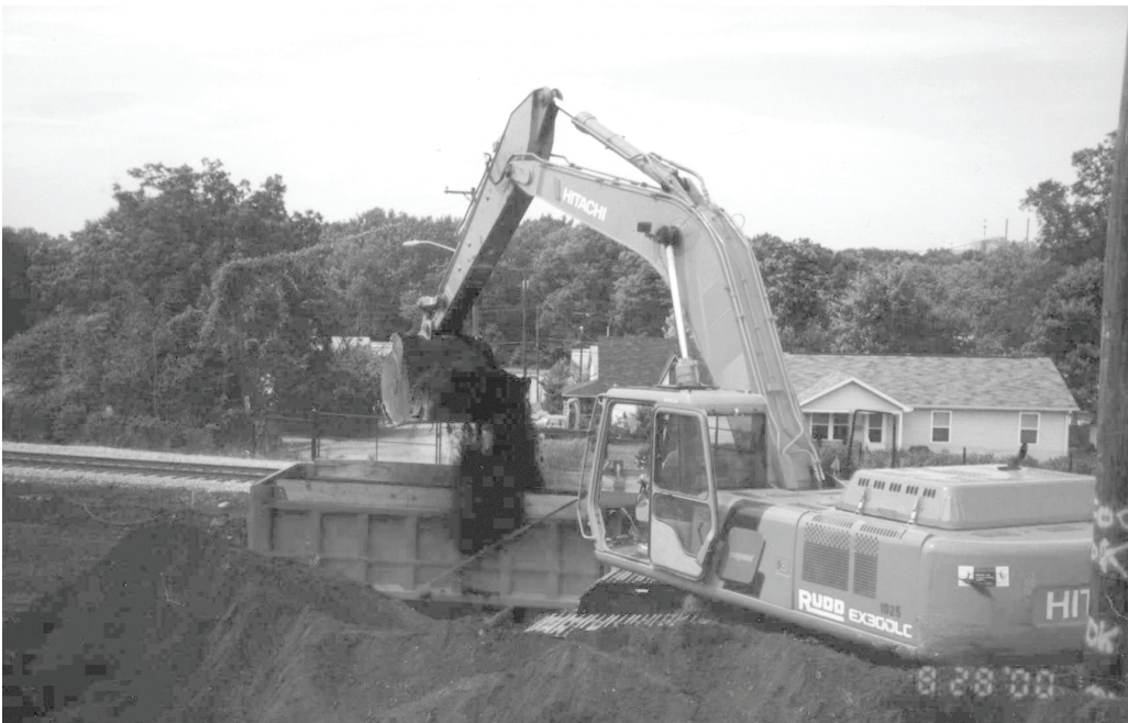
Figure 8-14. Track excavator loading trucks.
