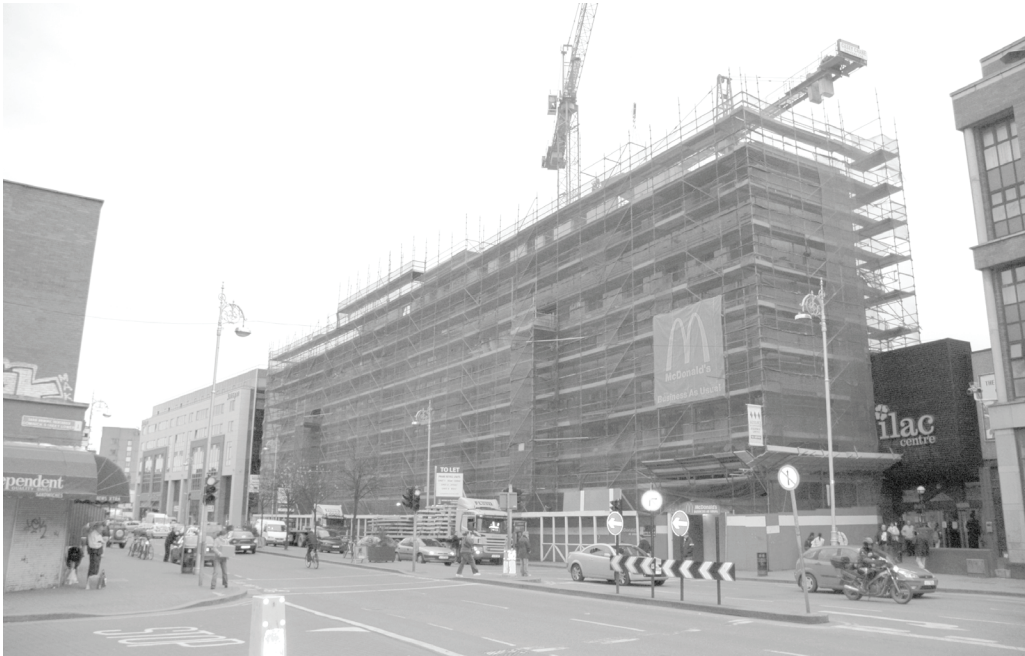
Figure 4-1. A typical site setup during construction.
