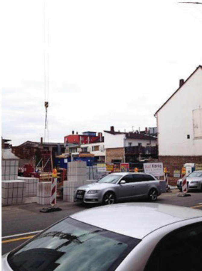
Figure 3-19. Construction site in Darmstadt, Germany, with multiple constraints: restricted site access, no easy locations for deliveries and materials handling, lack of temporary parking, and a clear need for road closures during construction.
