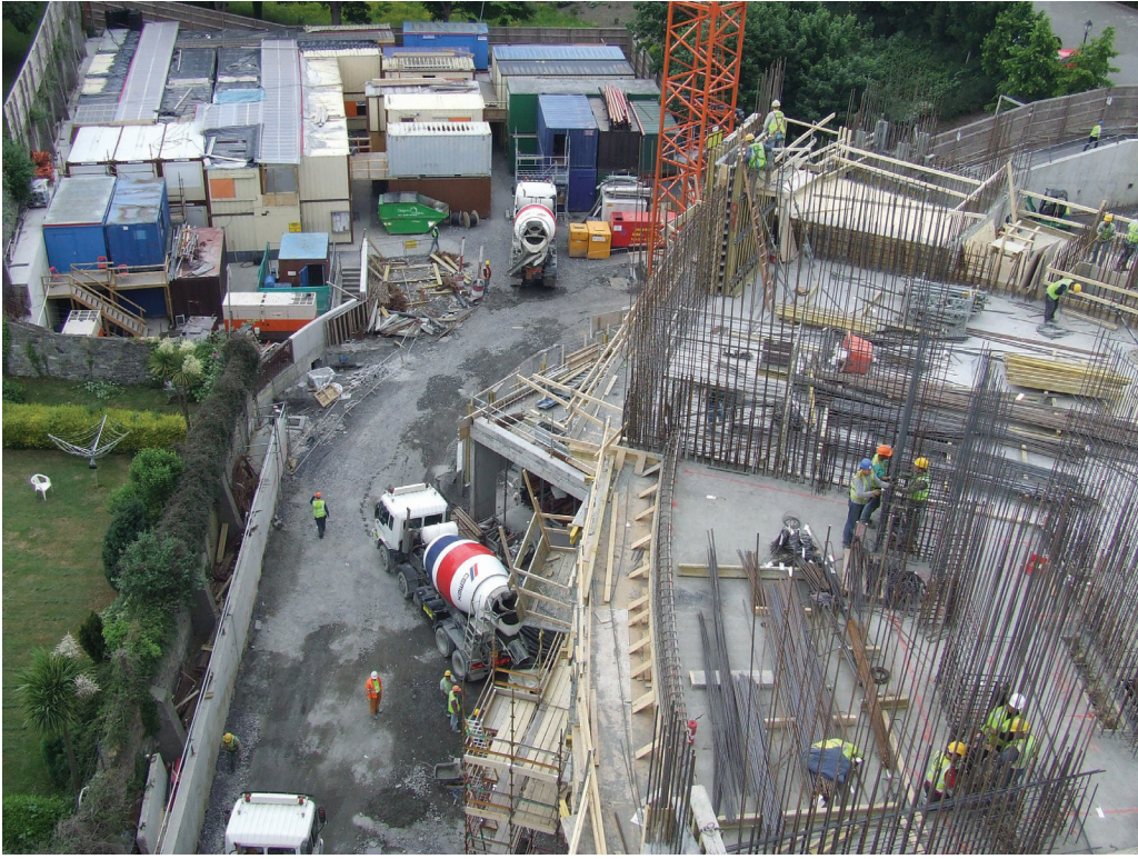
Figure 4-12. Typical site office layout on an Irish construction site.
