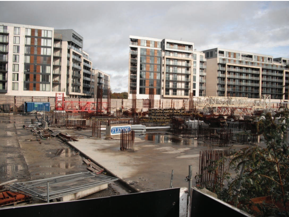
Figure 4-17. A building site during construction.
