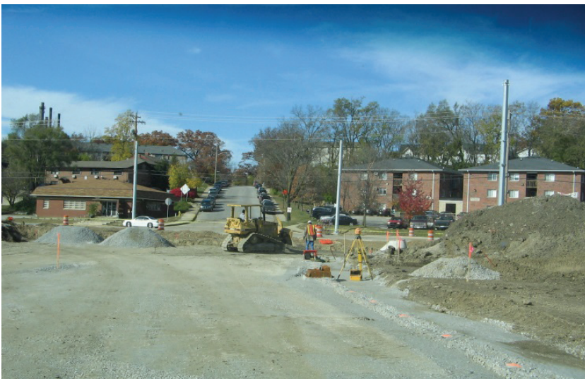
Figure 5-9. Checking grade with laser.
