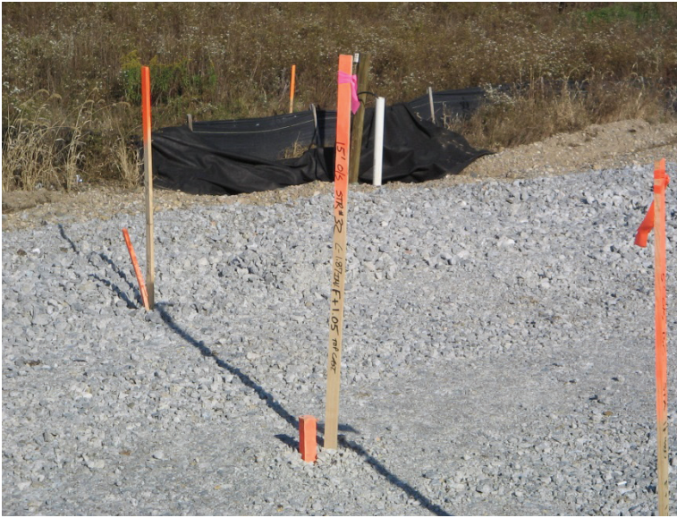
Figure 5-6. Drainage structure grade stake information to 0.01 ft.
