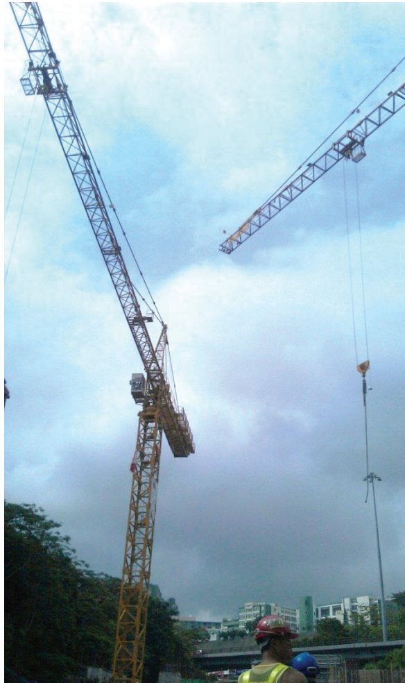
Figure 9-18. Tower cranes on a jobsite in China with collision monitoring.
