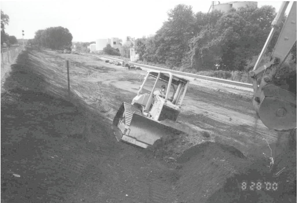
Figure 8-17. Dozer fine grading slope.
