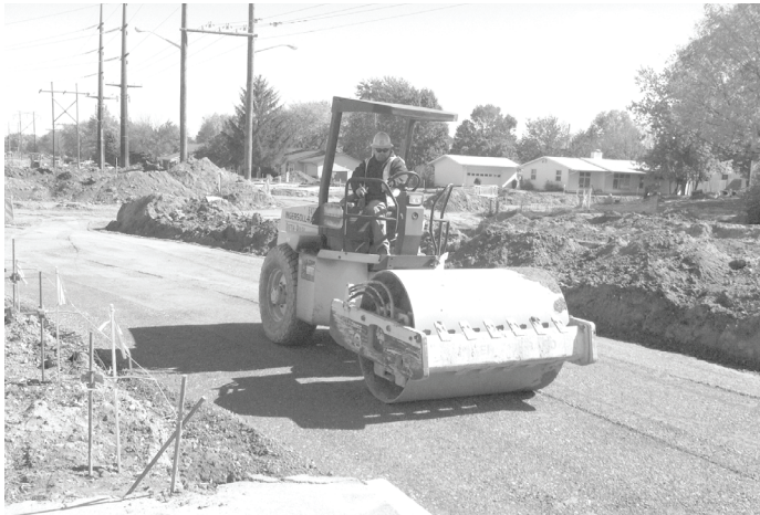
Figure 6-19. Compaction with smooth-wheel vibratory roller. This roller commonly compacts coarse-grained soils and rock fills.
