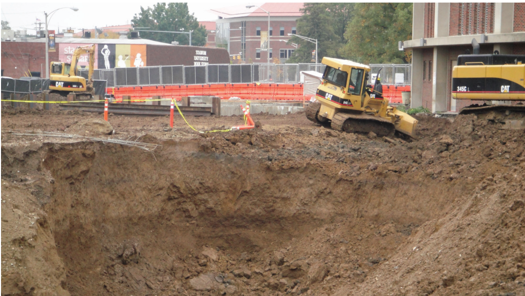
Figure 6-17. Vertical excavation of clay. Despite the initial stability of steep slopes, they must be cut back for safety to at least 0.75H:1V, and maybe more, if a soil retaining structure is not built.
