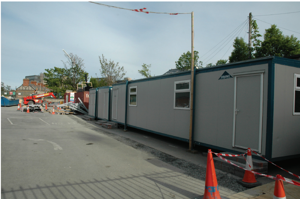
Figure 4-5. Typical site setup during construction on an Irish construction site.
