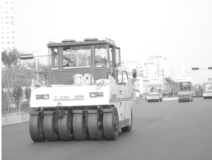
Figure 6-21. Pneumatic-tired roller compacting asphalt. Tire pressure can be regulated to obtain optimum results. This roller type can often be the most flexible for varied compaction requirements.
