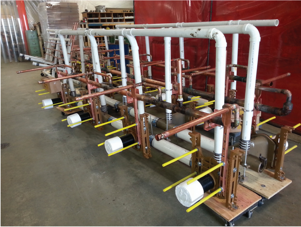
Figure 7-17. Prefabrication of commercial bathroom piping and supports.
