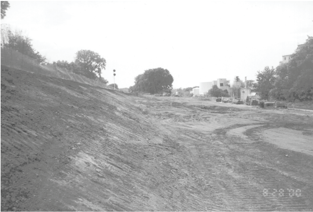
Figure 8-18. The finished product of a mass excavation that employed one track excavator set up to perform mass excavation, several haul units, a dozer designed to grade slopes, a dozer at the dump site (often forgotten in the estimate), and a foreman to manage to process.
