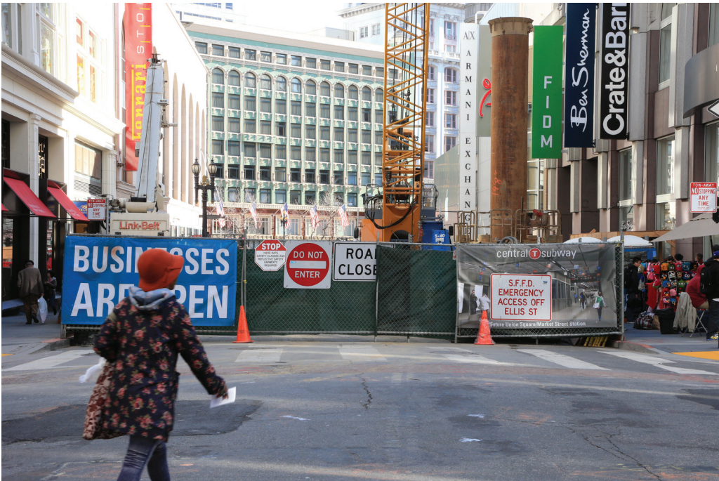
Figure 11-9. Site access is controlled by the use of signs and fences.
