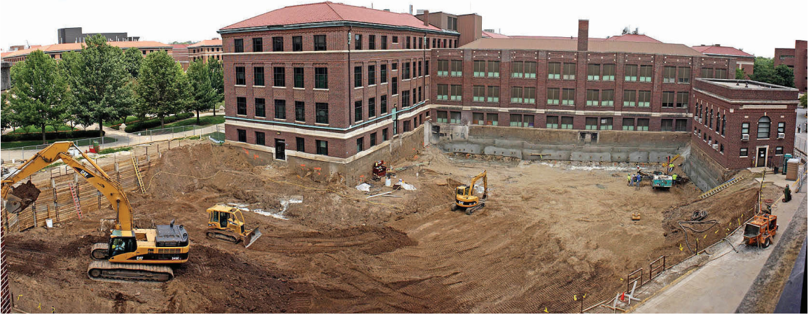
Figure 6-6. Earthwork at a building construction site.
