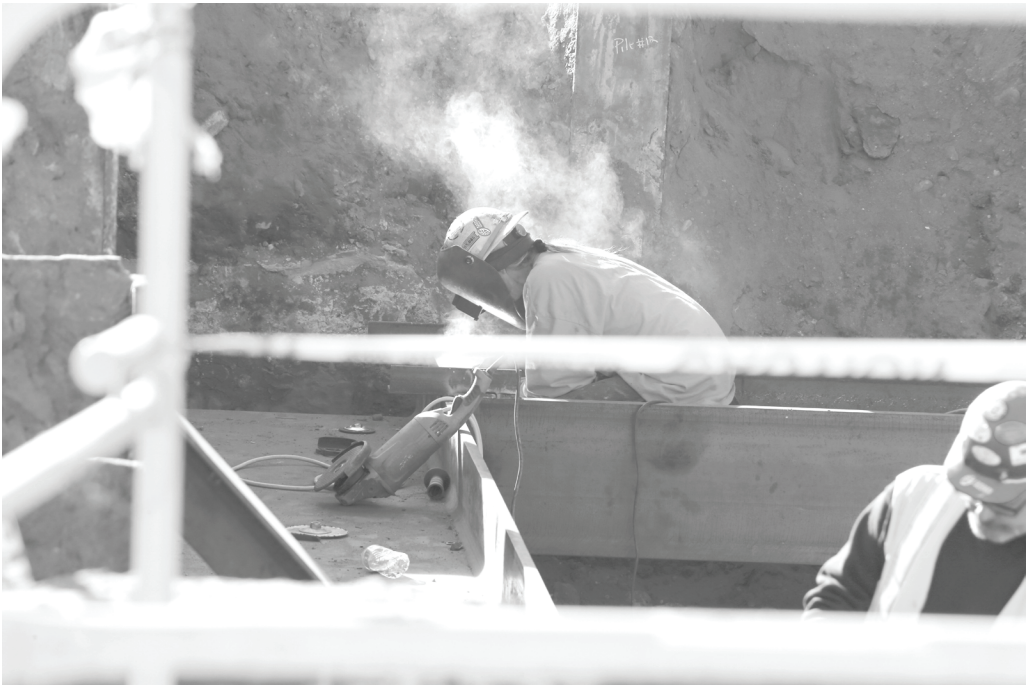
Figure 11-4. Face protection in use during welding operations.
