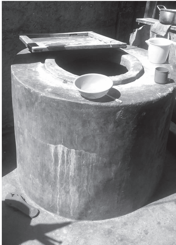
Figure 24.2 Cylindrical cement tank in Cariacó, Pemba.
