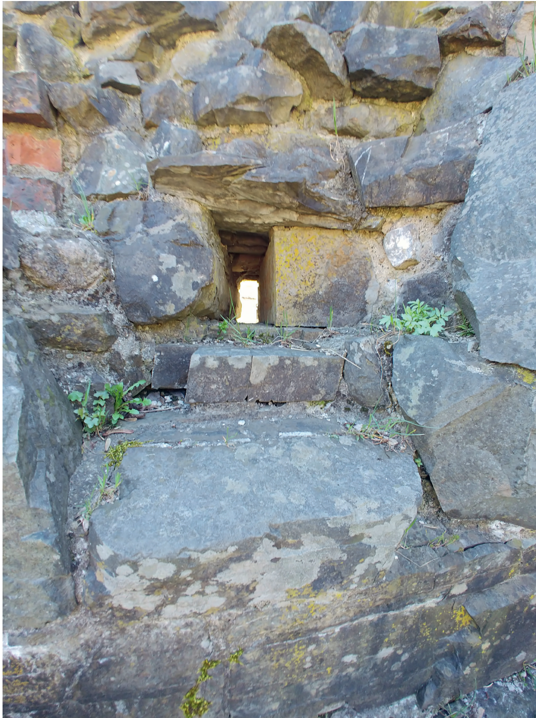
Figure 4. Basin and channel through the cloister wall in the kitchen at Hovedøya. Photo: M. Vedeler.
