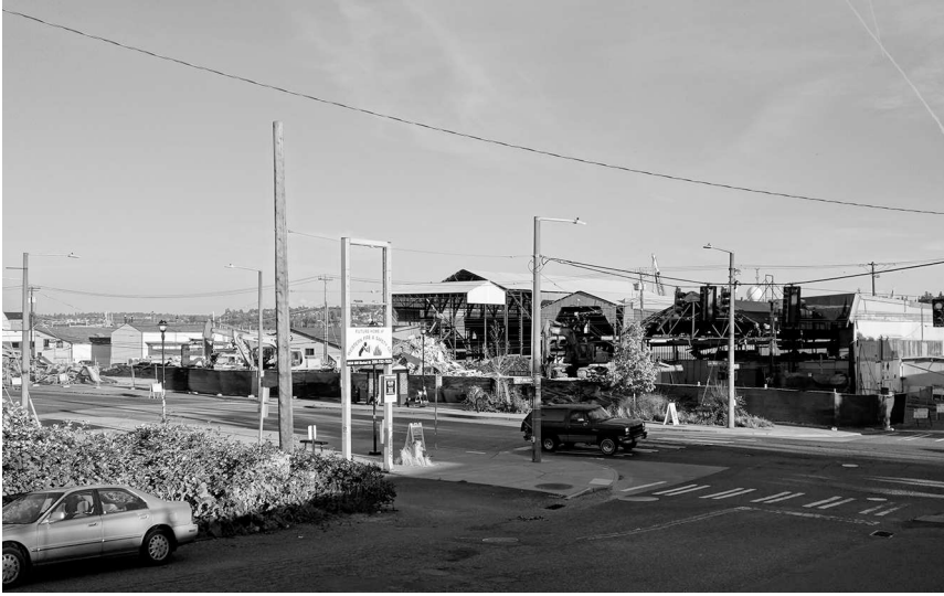
Figure 4.1 National Nordic Museum construction site in Ballard.
