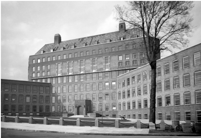
Fig. 1.7. The former WRNS Training Depot at Mill Hill shortly after its opening as the Headquarters of the Medical Research Council in 1950. Image courtesy of Associated Press/Alamy Stock Photo. https://www.alamy.com/medicines-back-room-boys-in-their-new-headquarters-at-mill-hill-london-on-march-21-1950-having-waited-ten-years-for-it-to-be-opened-due-to-the-war-the-building-was-used-by-the-admiralty-during-the-war-as-a-training-centre-for-wrns-the-exterior-of-the-new-building-which-will-house-the-research-workers-in-their-experiments-and-tests-ap-photo-image519356228.html
