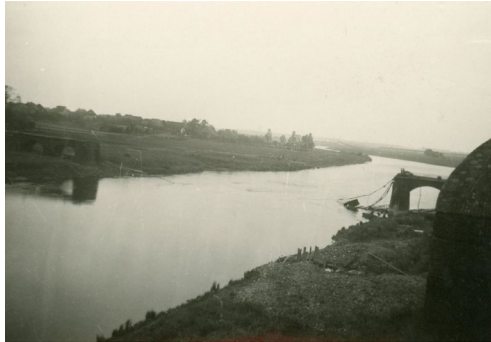
Fig. 6.27. Blown railway bridge across the River Weser, Minden, August 1945. Photograph by Joan Prior. Private papers of Joan Halverson Smith.
