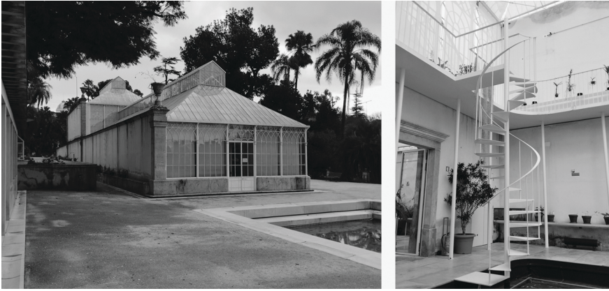
Figure 11.4 Coimbra Botanical Garden Tropical Greenhouses (2016), João Mendes Ribeiro architect. The first image shows the northern façade of the building and the side door on the central axis of the main route through the three naves. The second shows how the new elements, such as the spiral staircase, are integrated with the preexisting structural elements of the central nave.
