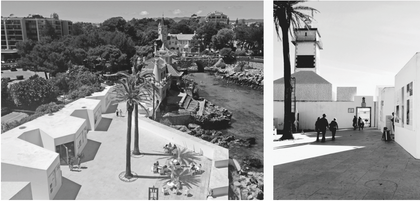
Figure 11.3 Conservation and extension of the Farol Museu de Santa Marta (2003–2007), architects. Manuel e Francisco Aires Mateus. The first image shows the new open space created in front of the inhabited “wall”, within a fortified enclosure and connected to the circuit of the Cascais Museum Quarter. The second image shows the entrance to the Lighthouse Museum.
