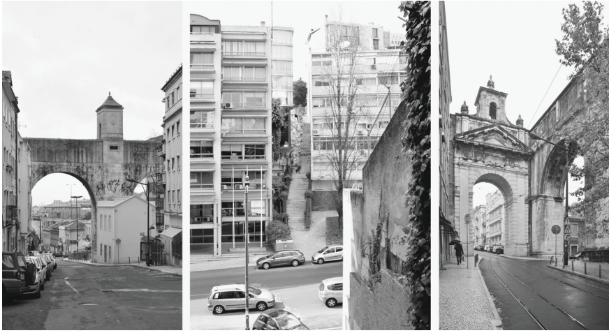
Figure 7.4 Back of the aqueduct intersection at Arco do Carvalhão with attached building (left). Ruins of the intersected aqueduct by Avenida Infante Santo (middle). Triumphal arch in Rua das Amoreiras (right).
