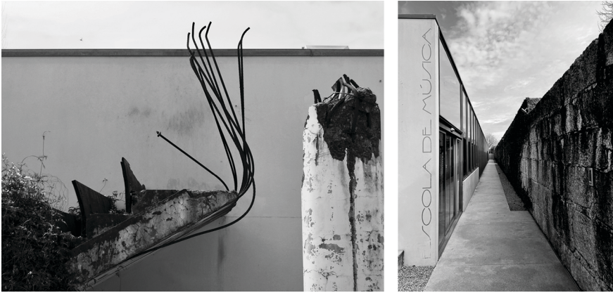
Figure 11.1 Conversion of the Braga market into a music school (2004–2010). The left photograph shows the remains of the stairs and columns that remained after the demolition of the market's roof. In their original design they were inspired by Greek stoas, and in their current state of ruin they reinforce this analogy with the project. The right image shows the main entrance of the Music School.
