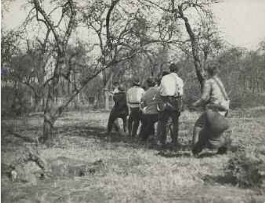
Fig. 16 Boys from the Polytechnic helped to clear the land at Chiswick in preparation for the new sports ground.
