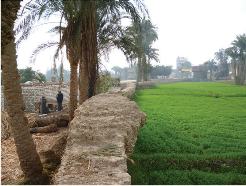
Figure 10. Remains of the Iṣā-ʿIzbat Abū al-Nūr dike near Iṣā. Photo by author, 2011.
