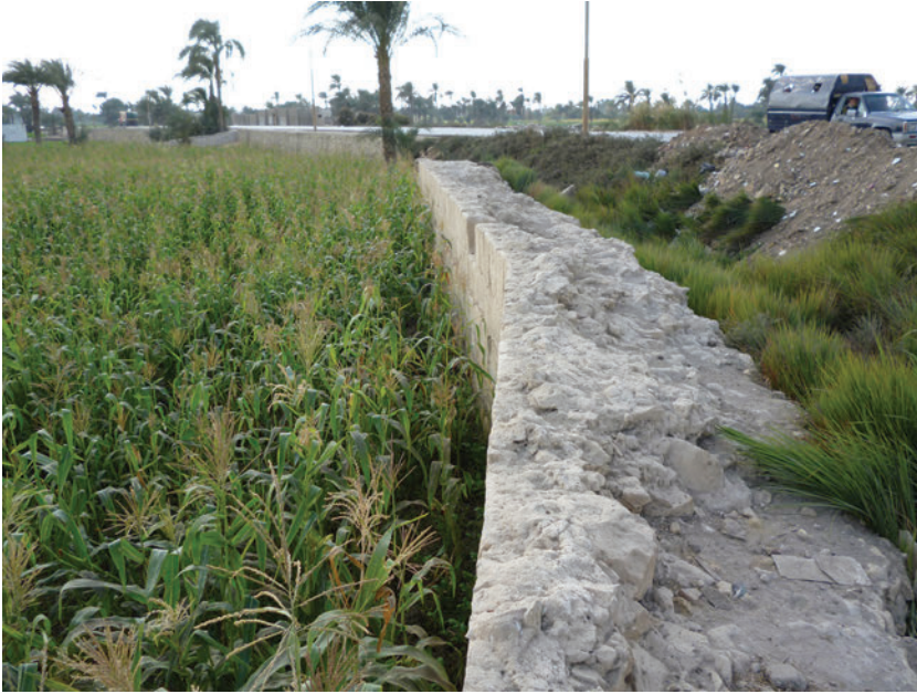
Figure 11. Stone-faced section of the Iṣṣā-‘Izbat Abū al-Nūr dike near Iṣṣā. Photo by author, 2011.
