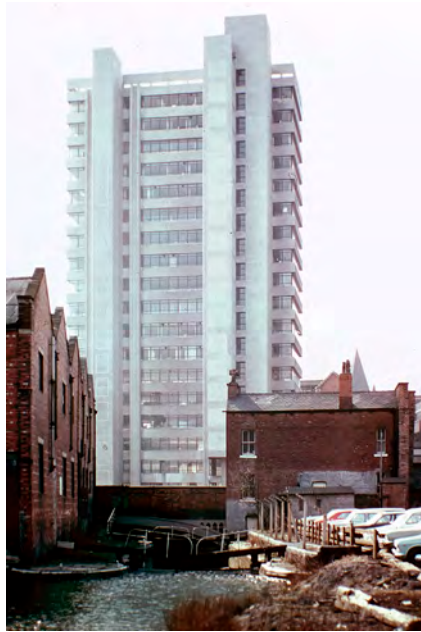
Figure 4.01 Rodwell House (Douglas Stephen & Partners, 1965). The base of the building straddles the Rochdale Canal, which runs beneath it.
