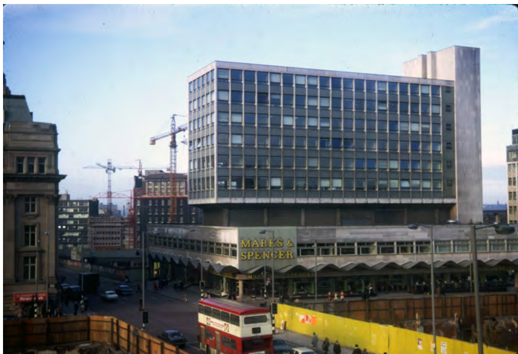
Figure 5.12 Michael House and Marks & Spencer. To the rear the cranes for the further development of Market Place can be seen. In the foreground are the hoardings around the site of the Arndale Shopping Centre.
