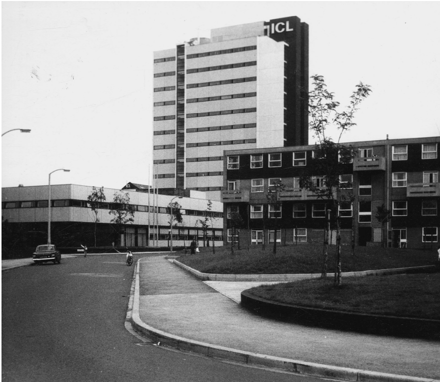
Figure 2.19 Gorton, Wenlock Way off Clover Street, ICL in view, flats. The brave new world of late 1960s Manchester and the reinvestment in east Manchester is evident in this composition that appears to deliberately situate new housing and industry side by side – the new terrace. The low block to the left of the image housed the research department.
