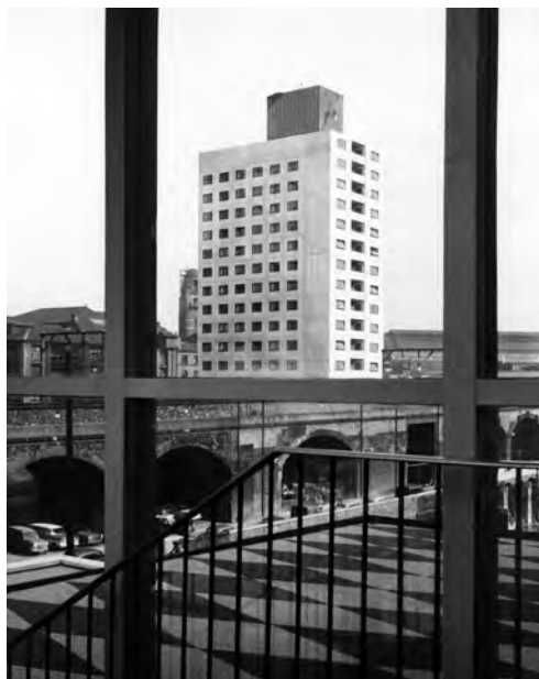
Figure 3.16 Chandos Hall viewed from the stairwell of the Renold Building.
