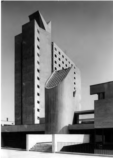
Figure 3.19 The stair and lift tower of Wright Robinson Hall.
