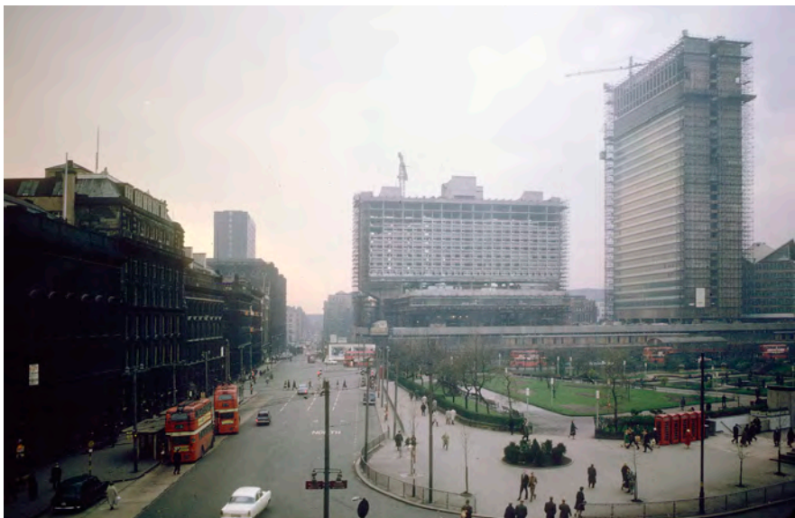
Figure 6.18 Piccadilly Plaza under construction. The smog-laden haze and soot-blackened Victorian buildings testify to the city's industrial roots.
