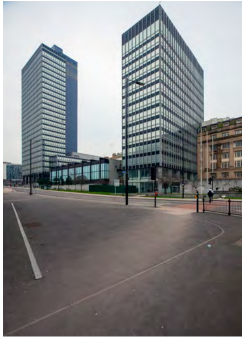
Figure 6.15 CWS and CIS Towers.
