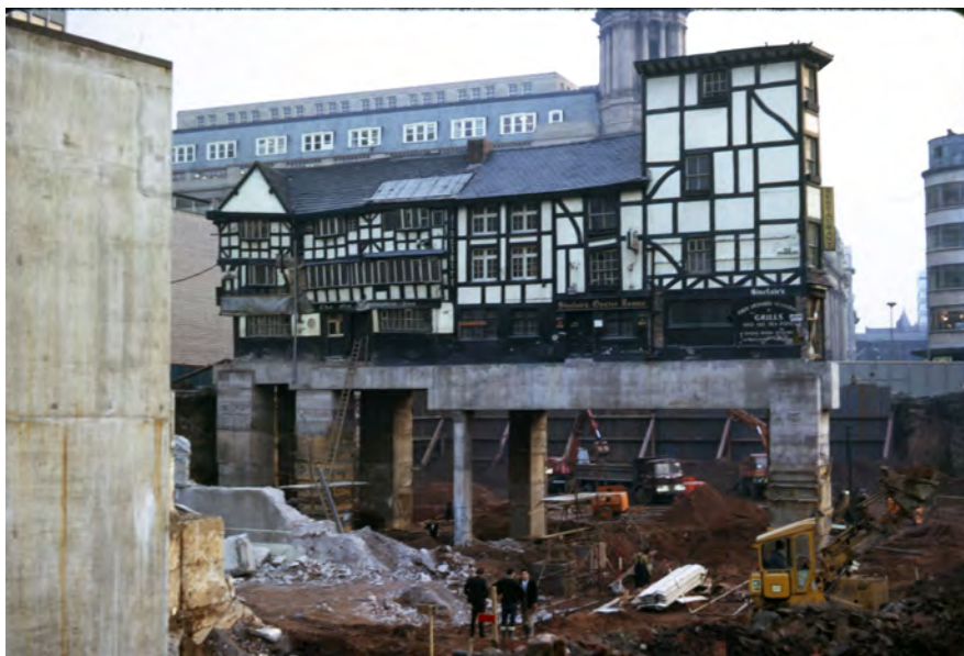
Figure 5.16 The Shambles being lifted up. The Old Wellington Inn (left) and Sinclair's Oyster Bar (right) elevated on concrete stilts during the construction process to meet the new datum established as part of the city centre stratification and separation of cars and pedestrians.
