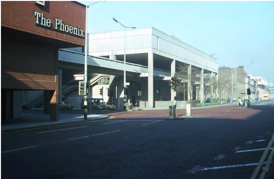
Figure 3.32 Bridge connecting the Precinct Centre to the RNCM.
