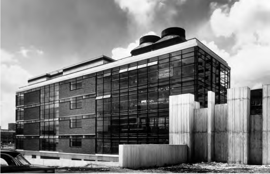
Figure 3.23 Chemical Engineering Pilot Plant.
