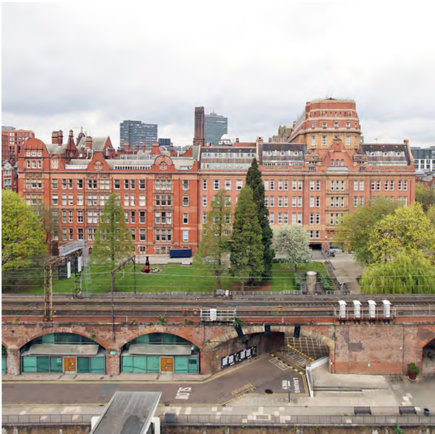
Figure 3.03 The Sackville Street Building viewed from the top floor of the Renold Building. The original building is to the left and the extension to the right.
