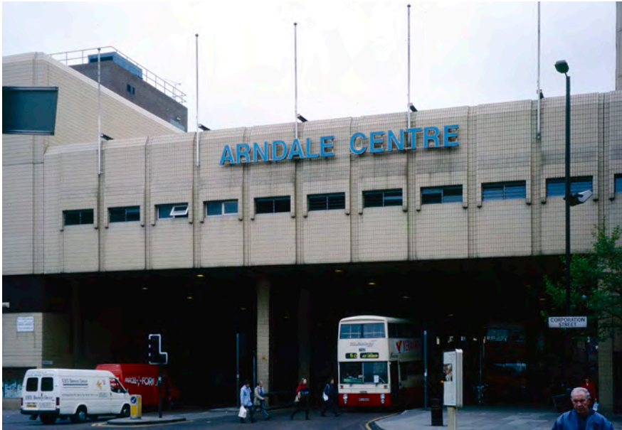
Figure 5.30 The Arndale Centre, Wilson & Womersley, 1977.
