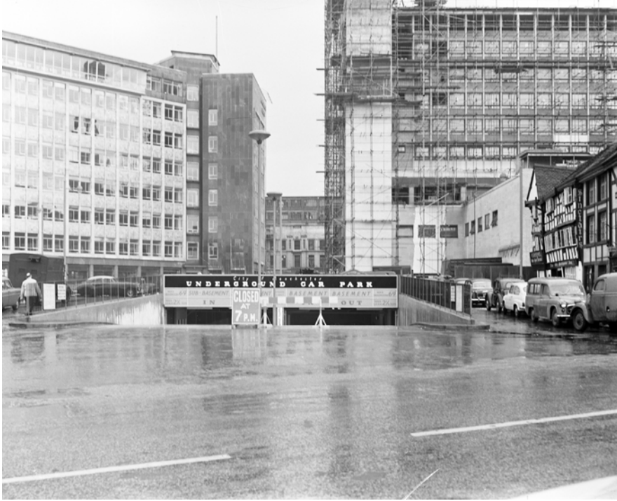
Figure 5.10 Entrance to the Corporation's underground car park. In the right foreground are the Old Wellington and Sinclair's. In the background on the left is Longridge House and on the right Michael House is under construction.
