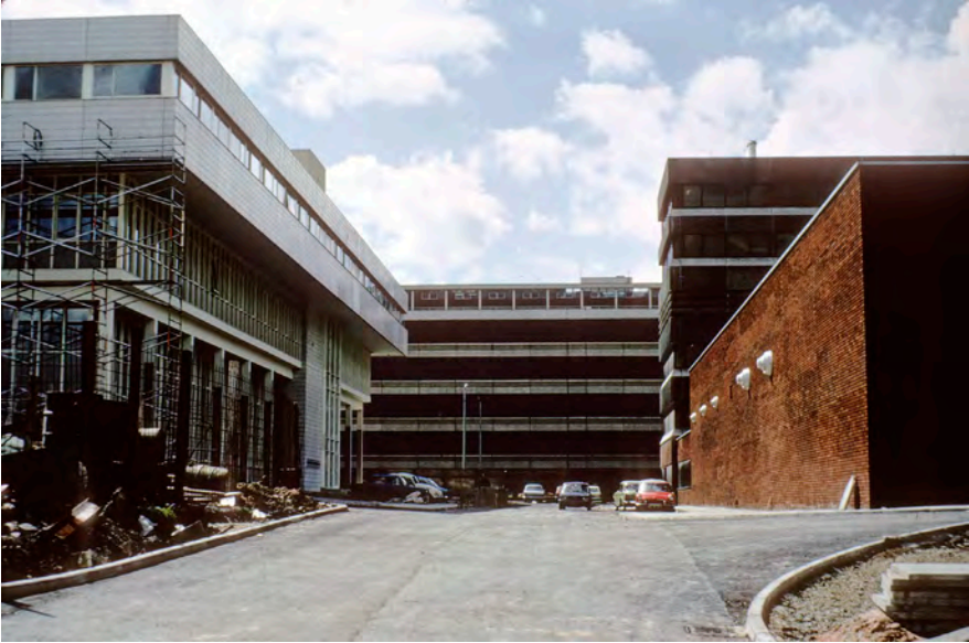
Figure 2.24 Photograph taken from between the National Computing Centre, Cruickshank & Seward, 1967–74 (left) and the BBC North headquarters, R.A. Sparkes, 1971–75 (right), looking across Oxford Road to the recently completed Phase II of the Municipal College of Technology (later Manchester Polytechnic), W.B. Heppell, City Architect, 1974.
