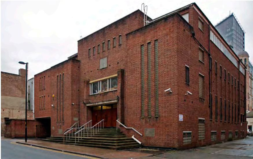
Figure 1.13 Manchester Reform Synagogue, Cummings & Levy, 1953, on Jackson's Row in the city centre.
