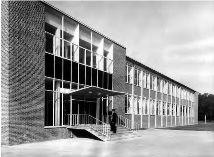
Figure 2.07 Entrance canopy to the Ferranti facility. The simple concrete frame with brick infill panels was common to several early buildings designed by Arthur Gibbon for Cruickshank & Seward.
