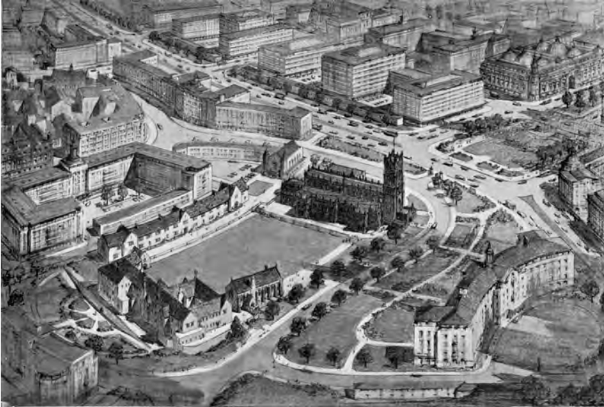
Figure 5.07 Drawing by P.D. Hepworth of the Cathedral Precinct. Above the Cathedral are shown the first illustrations of the new Market Place, a rectangular road junction and a series of orthogonal commercial blocks.
