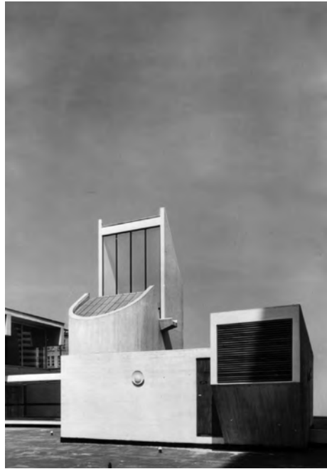
Figure 3.20 Expressive volumes on the roofscape of the Barnes Wallis Building.
