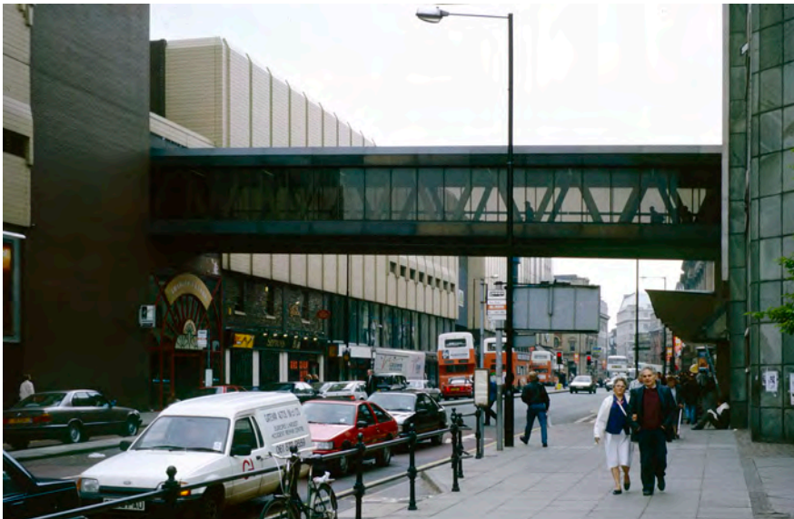
Figure 5.28 Footbridge connecting St Michael House to the Arndale Centre. It was destroyed in the 1996 IRA bombing and replaced by a new bridge designed by Stephen Hodder.
