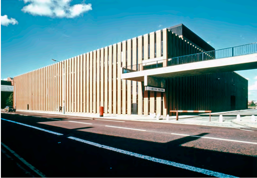
Figure 3.30 The upper-level entrance to the Kilburn Building (Computing) via a bridge link from the head of the ramp to the Maths Tower.
