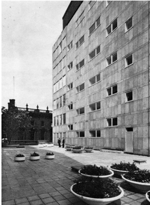
Figure 6.19 The roof garden of Williams Deacon Bank.
