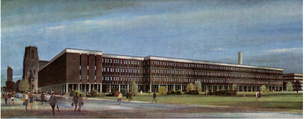
Figure 3.33 Artist's illustration of the long facade of the Medical School (H.S. Fairhurst & Sons, 1972–74). The soft landscaped area in front was reserved for the path of the inner ring road that was never constructed.
