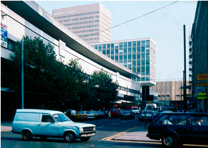
Figure 5.24 View eastwards along St Mary’s Gate from Deansgate, 1980. The strong horizontal banding and the set back upper floor and extended canopy were typical motifs in Cruickshank & Seward’s commercial work. In the background are Michael House and the buff-coloured tiles of the Arndale Centre and tower.
