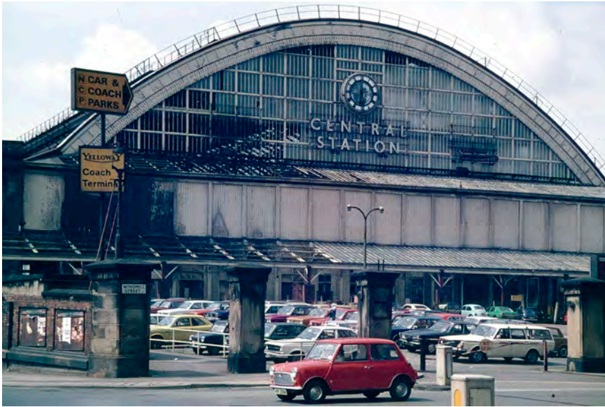
Figure 4.03 Central Station looking rather forlorn in 1975 after its closure in 1968 and its use predominantly as a car park in the intervening years.
