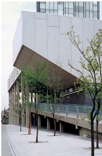
Figure 3.29 Ramped approach to the entrance of the Maths Tower, with the sloping soffit of the lecture theatre providing cursory shelter.
