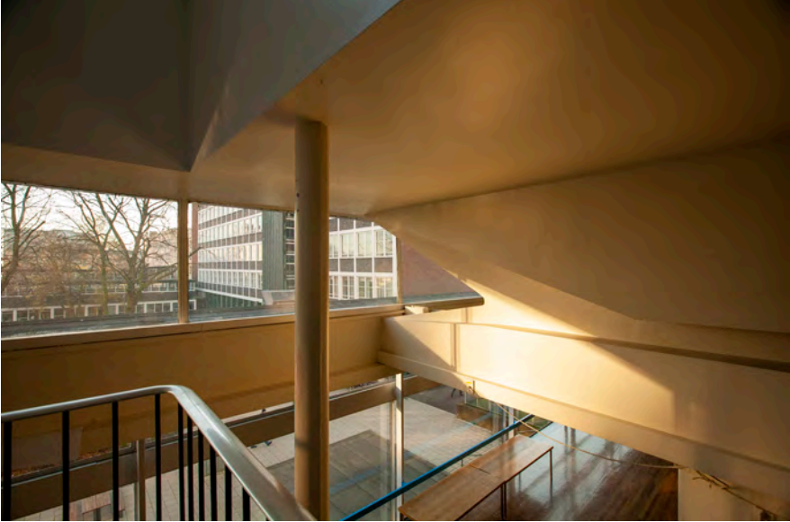
Figure 3.15 Bird's-mouth beams and open staircase.
