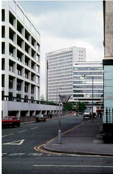
Figure 1.23 Viewed from Quay Street, the white gridded exoskeleton of the Magistrates' Court (Yorke Rosenberg Mardell with City Architect S.G. Besant Roberts, 1971) is on the left of this image. In the background can be seen the squat tower of Manchester House (Leach Rhodes Walker, 1965) and behind that, the Portland stone clad home of the inland revenue, Albert Bridge House (E.H. Banks, Ministry of Works, 1959).
