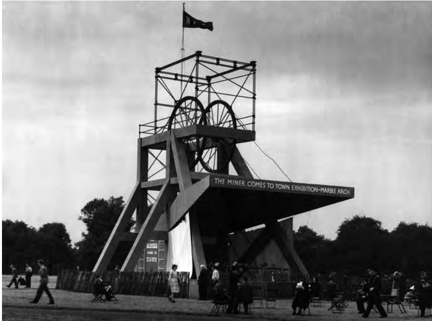
8.3 The Miner Comes to Town , organised by the Central Office of Information, designed by Peter Moro and Robin Day. Alfred Cracknell. Image courtesy of Architectural Press Archive / RIBA Collections. All rights reserved and permission to use the figure must be obtained from the copyright holder.
