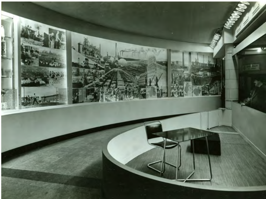
2.8 Do Not Pass by the Special Areas , Charing Cross Station, planned and designed by F. C. Pritchard, Wood & Partners. 1983/4/4333 © TfL from the London Transport Museum collection. All rights reserved and permission to use the figure must be obtained from the copyright holder.
