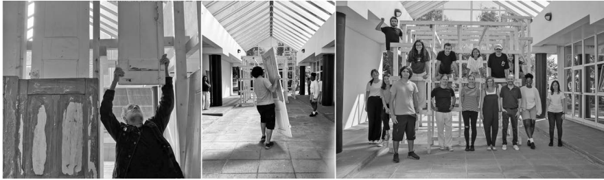
Figure 12.4 ADAPT workshop – Participatory hands-on process of construction.
