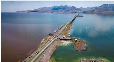
Urmia Lake Bridge
