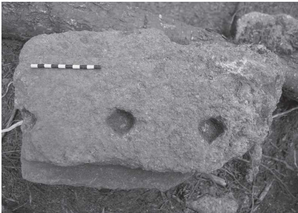
Figure 12.14. Window masonry showing holes made for iron bars.
