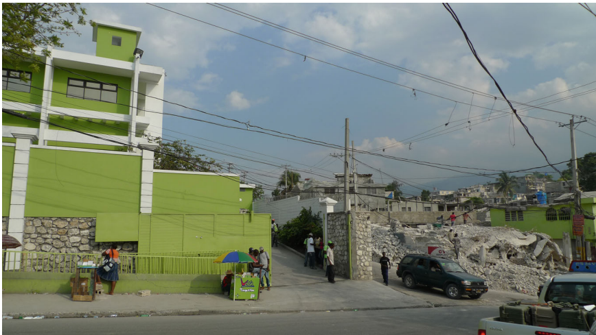
Fig. 3.1 During the 2010 Haiti earthquake the well-built commercial building on the left sustained no damage, and non-structural effects commensurate with MMI V. The building on the right collapsed catastrophically
