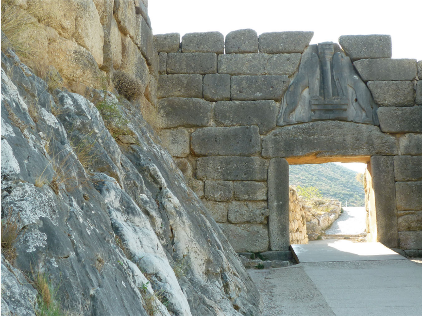
Fig. 4.9 The world-famous Lion Gate at Mycenaean (Greece). The fortification wall was built on top of an active, Aegean-type, limestone fault scarp (see Stewart and Hancock 1988 for further reading), eliciting the question whether or not Mycenaean were aware of the earthquake hazard threatening their city
