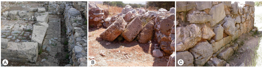
Fig. 4.6 Examples of secondary structural PEAEs in archaeological contexts dominated by rubble architecture. (A) Tilted base of wall at Amnisos (Crete, Greece). (B) Domino-type collapsed wall segment at Malia (Crete, Greece). (C) Rotated block in a wall at Zakros (Crete, Greece). Compared to equivalent secondary structural PEAEs in monumental masonry constructions (Fig. 4), proving an earthquake hypothesis in these rubble contexts remains very challenging
