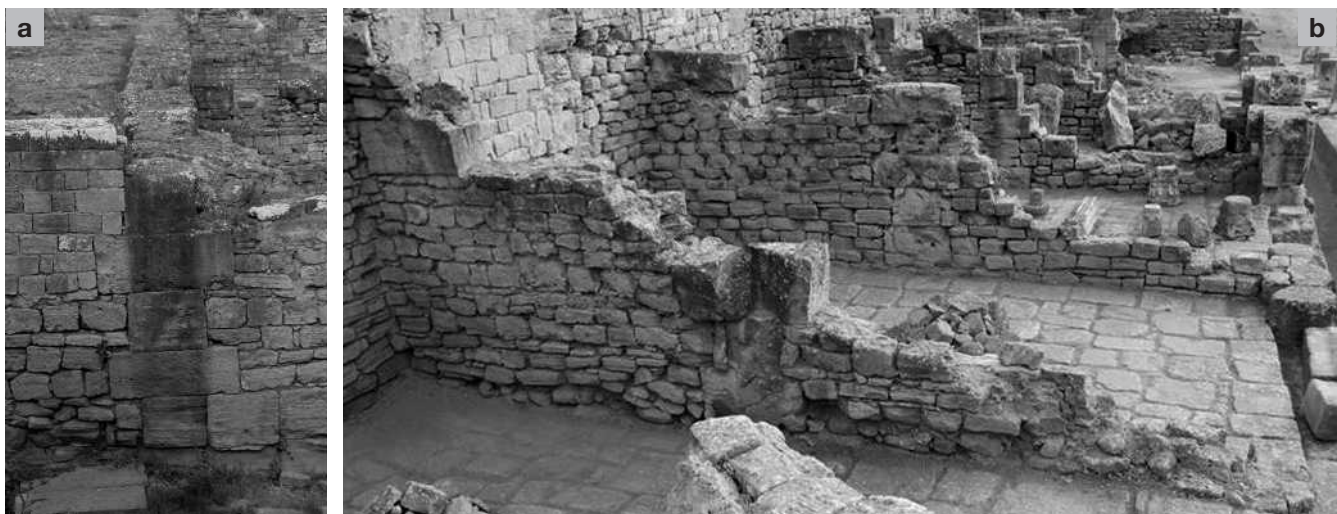
Figure 5.9. Capitulum of Sala: position and function of the piers. A: links between perpendicular walls; B: points where the weight of the south colonnade discharged on the vaults of the tabernae (photos: S. Camporeale).
