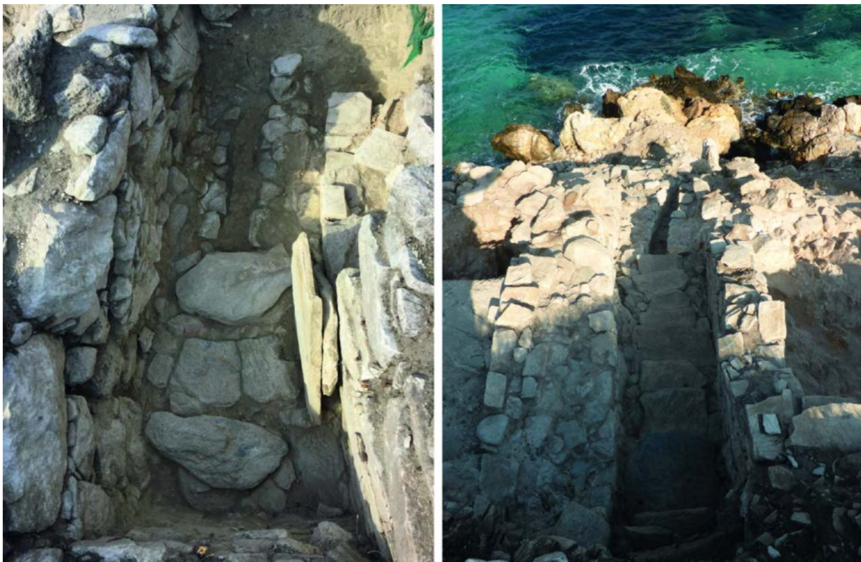
Fig. 2 – Drainage systems under the streets of Dhaskalio. – (Photo: Keros Project).
