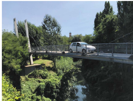
Figure 4.34: Test of the bridge using a small car as load.
