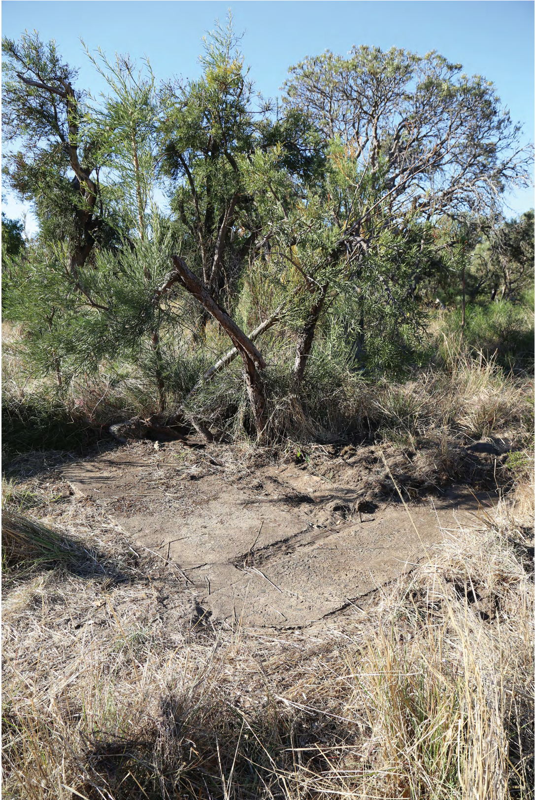
Figure 12.10. Concrete pad, inset wooden supports and borehole.
