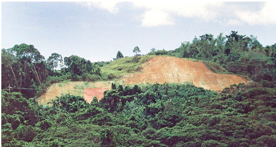
Figure 7.6. Section where the Compact Road has cut through east side of the Ngebars earthworks in Ngatpang.
