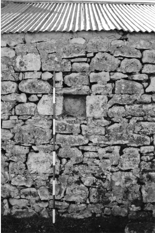
Figure 10.4. Exterior of extant embrasure in the ‘men’s hut’ at Central Outstation, subsequently blocked up.
