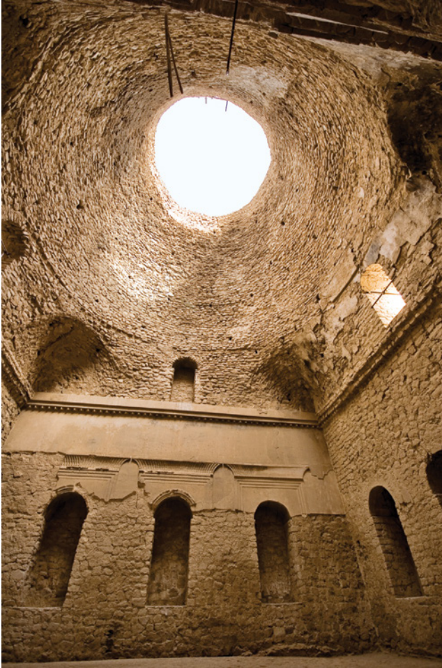
FIGURE 11.8 Throne room at the palace of Ardashir I, Firuzabad. Square room with a domed roof executed in pitched courses of mudbrick.
