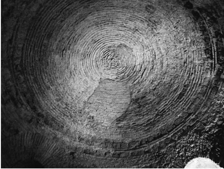
FIGURE 11.13 Pitched brick dome in a basement room of the residential apartments, Diocletian's palace, Split. The technique of executing domes with pitched courses of brick is unknown in imperial architecture before the Tetrarchic period and probably came to the Roman Empire from the east. AUTHOR'S PHOTOGRAPH.
