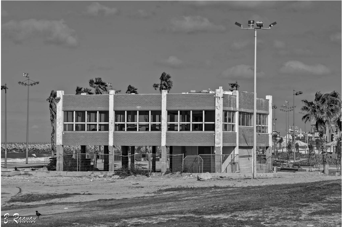
Figure 15.7 “Kiosk” at Lido Beach, Ashdod, after illegal extension demolished
