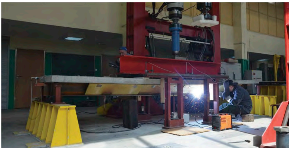
Figure 4. Welding of a strengthening plate.
