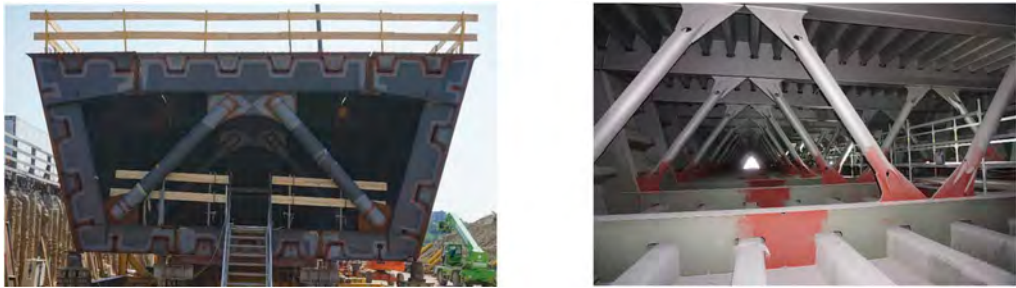
Figure 1. Design variants of tubular bracing inside of box girders of the German bridges Heidingsfeld (left) and Schierstein (right) (Kuhlmann & Gözl 2021).
