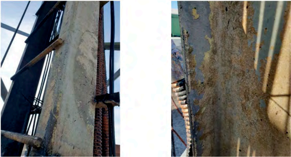
Figure 6. The effect of elevated temperature on components of the ladder rails (D-8 element).
