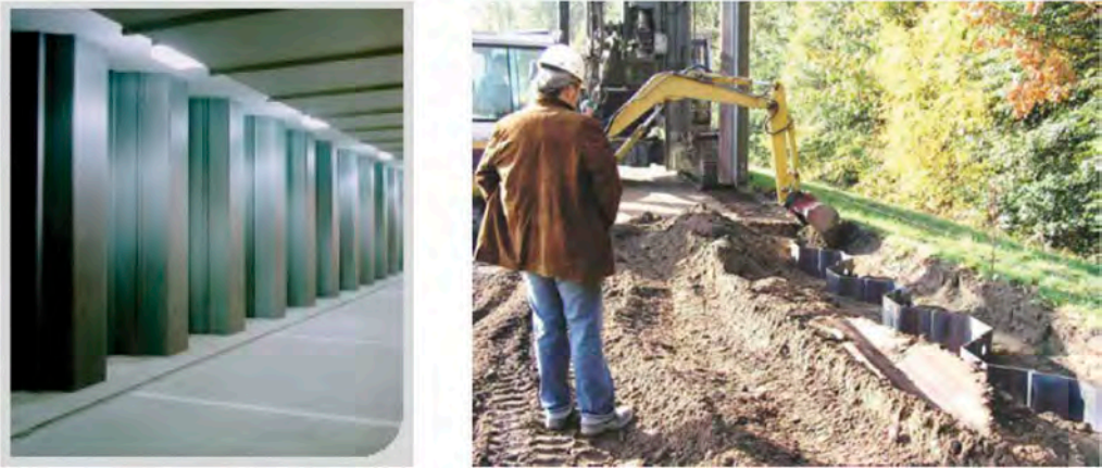
Figure 1. Examples of U sheet pile wall.
