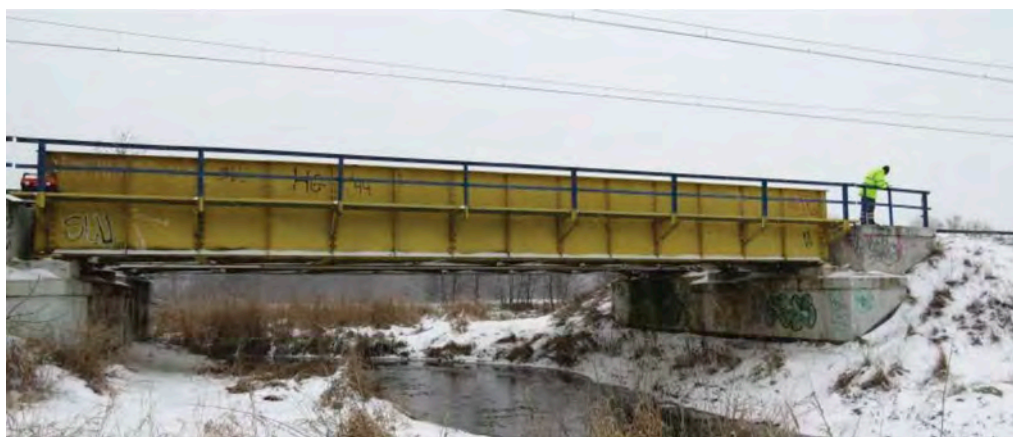
Figure 1. View of the span of the railroad bridge on km 207.887 of the railway line No. 7 Warszawa Wschodnia – Dorohusk.
