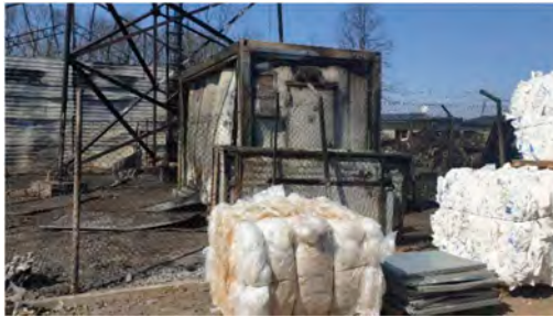
Figure 5. The telecom shelter destroyed during the incident.
