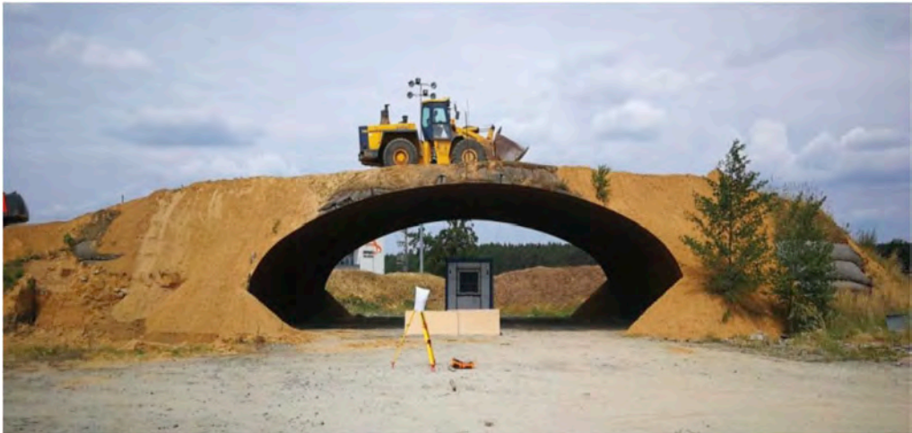
Figure 1. View of the loaded structure.
