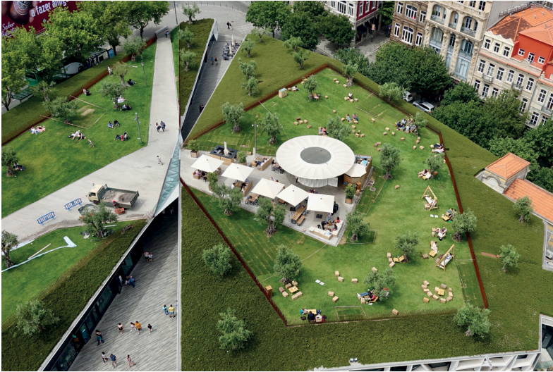
Figure 6.6 Porto's Praça de Lisboa now contains a new high-level park (above retail and parking) in the centre of an area formerly in decline. The site was subject to two competitions organised respectively by the municipality and by a citizens' collective who launched the 'No rules, great spot' competition to encourage debate about the future of the space. The final scheme was carefully controlled, being immediately adjacent to the boundary of the UNESCO World Heritage site, yet establishes an innovative green space within which relaxed informal activities occur with users shaping the space daily to their own ends (image: Matthew Carmona).
