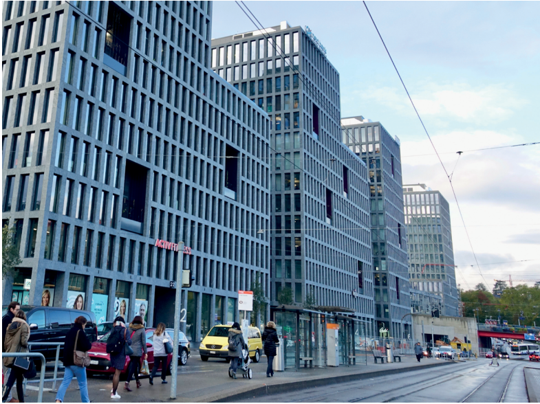
Figure 6.4 In Geneva, the need to build new housing to tackle an affordability crisis has led to major expansion plans, including here in the huge Acacias Bâtie redevelopment area. This has been accompanied by a realisation that major growth needs to be underpinned by a consistent emphasis on high-quality Baukultur , something that has not always been the case in the past (image: Matthew Carmona).
