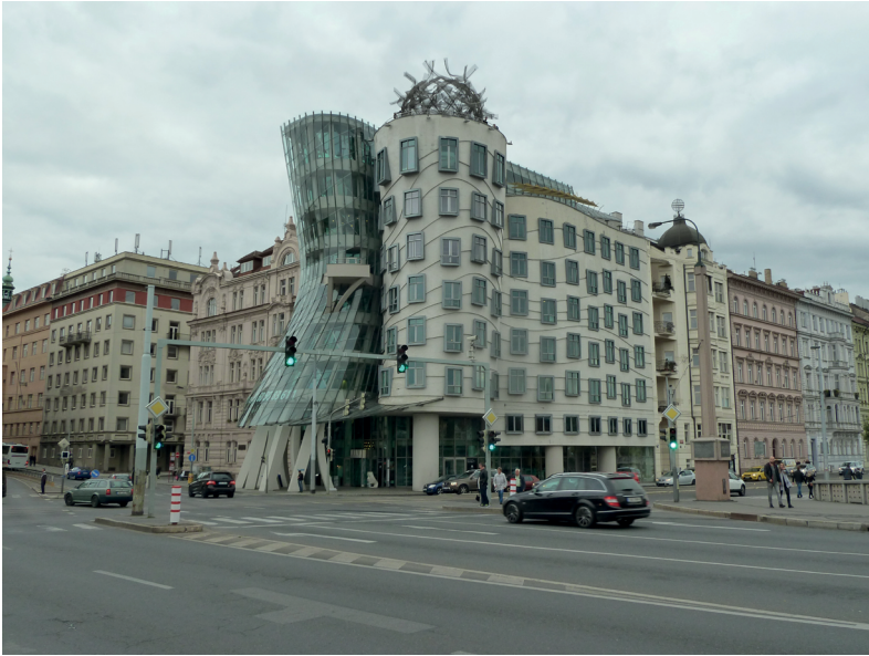
Figure 2.2 Frank Gehry's Dancing House in Prague, completed in 1996, draws praise and criticism in equal measure. It is clearly a creative and very contemporary building in a historic setting, but while it contrasts with its surroundings, it also fits in through the use of materials, proportions, and height and massing parameters that respects its neighbours. In this case not only did the site create its own constraints, but so also did the fixed zoning system of Czech cities where development quantum and heights are controlled; in this case courtesy of the Plan of the Stabilized Zones of Prague , produced by the Chief Architect's Office (prior to the abolition of that position) in 1994 in order to guide the post-communist restructuring of the already built-up sections of the city (image: Matthew Carmona).
