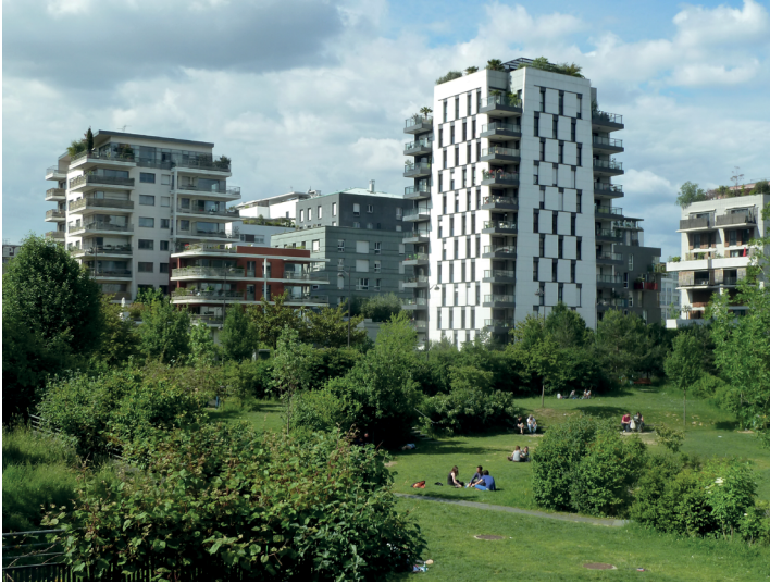
Figure 4.28 The observatory of the architectural quality of housing, collected by the Île-de-France association, provides learning from regionally significant projects such as the Quartier Massena in Paris (image: Matthew Carmona).
