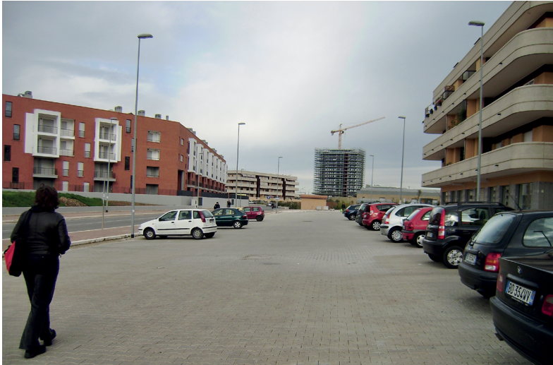
Figure 1.4 Different developers have constructed standard apartment block types on both sides of this street in Rome, applying a standard road and footpath typology. Height and set-back controls have been respected but provision of parking (on the left in a podium creating a blank frontage onto the footpath, and on the right in a relentlessly hard street-level parking area) undermines any quality in the public realm (image: Matthew Carmona).
