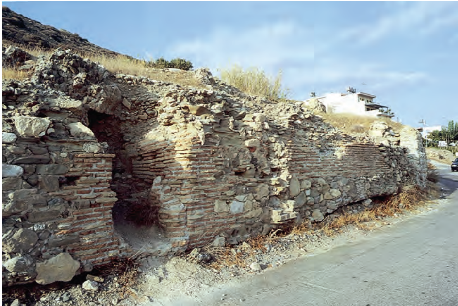
Plate 2 Myrtos: road-cut exposing hypocaustal brick (photographer facing north-east)
