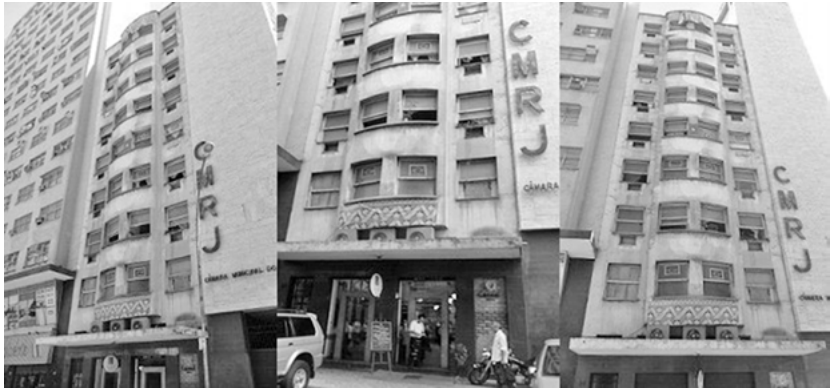
Figure 9: Front view of Manoel Congo 81
