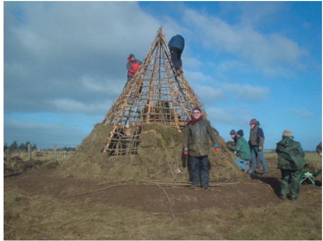
Figure 13.11 Despite initial concerns the turf stayed in place and was made secure by using twists of willow to peg them over the underlying lattice.
