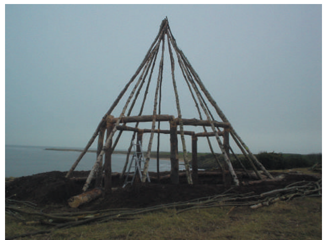
Figure 13.8 Construction 2 used long slender roofing poles made from birch providing a steep pitch around 60°
