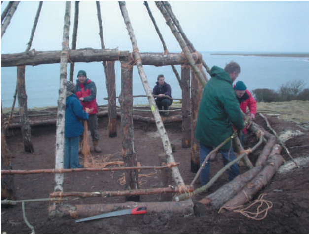
Figure 13.9 The birch pole superstructure gained immense stability once the spars were tied across them.
