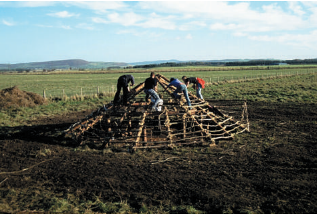
Figure 13.4 Lashing the coppiced poles (purlins) on to the timber frame.
