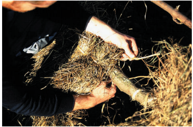
Figure 13.6 Detailed view of lashing the thatch on to the purlins using plant fibre cord.
