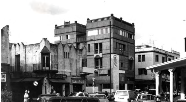
Figure 10.2 Sotiris Koukis, office building in the Athenian apartment building typology, Rhodes, 1968 (top), transformed into the local branch of the Ionian Bank by Suzana and Dimitris Antonakakis, 1986 (bottom) Suzana and Dimitris Antonakakis' private archive
