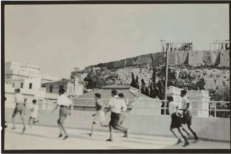
Figure 6.4 Patroklos Karantinos, School on Kalisperi Street under the Acropolis in Athens, 1931–2, photographed by Sigfried Giedion in August 1933
