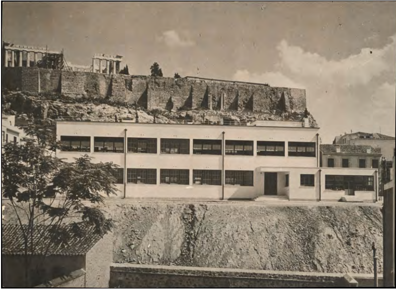
Figure 6.3 Patroklos Karantinos, School on Kalisperi Street under the Acropolis in Athens, 1931–2, south elevation, unknown photographer Andreas Giacumacatos's private archive
