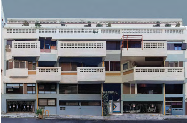
Figure 9.16 Suzana Antonakaki, apartment building on 44 Doxapatri Street, Athens, 1978–82, photographed by Dimitris Antonakakis and Sarra Matsa, 2021
