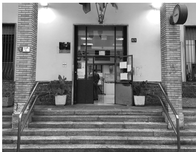
FIGURE 21.4 Casa Jannacci: The entrance. Source: Massimo Bricocoli, 2019.
