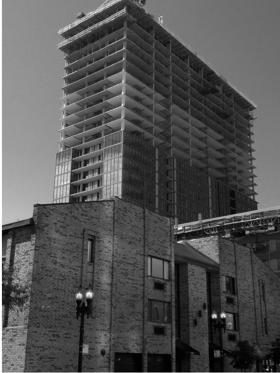
FIGURE 13.5 Old Town Park under construction.
