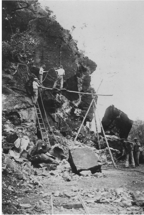
Figure 9 Digging a tunnel (Private collection)
