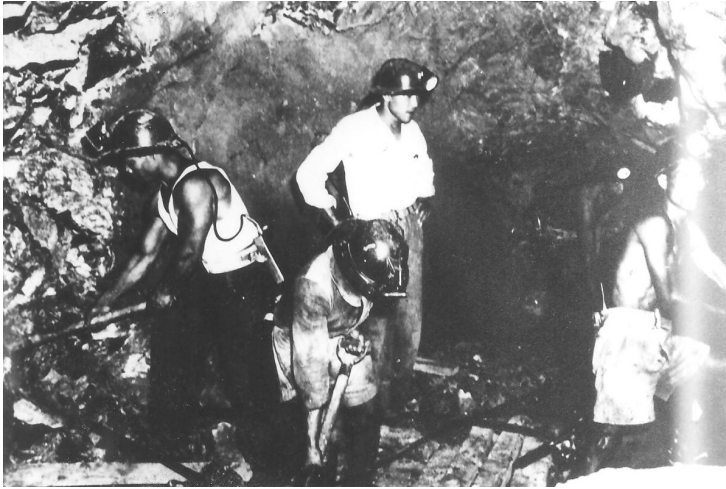
Figure 8 Underground chrome mine gallery (Private collection)
